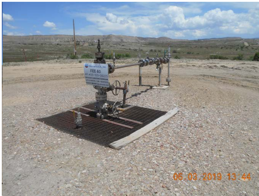
Injection wellhead.
