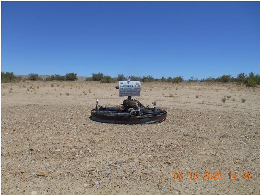
Injection wellhead. Temporarily Abandoned.
