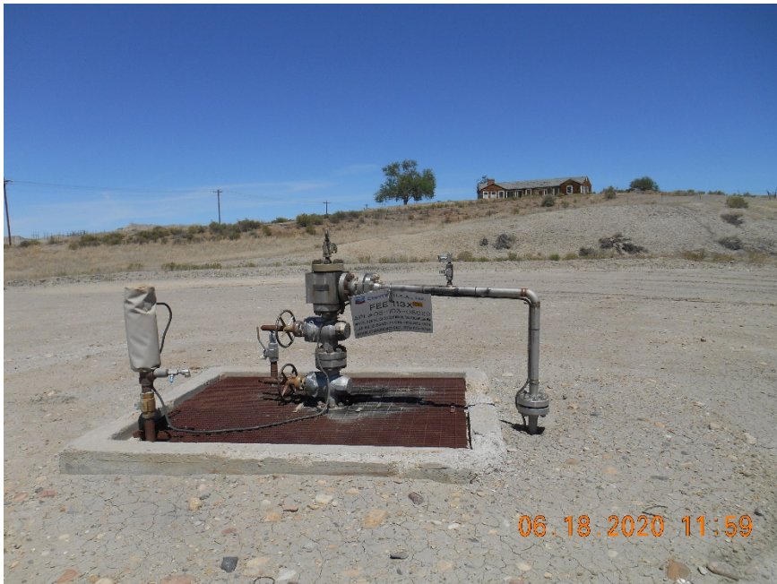
Injection wellhead
