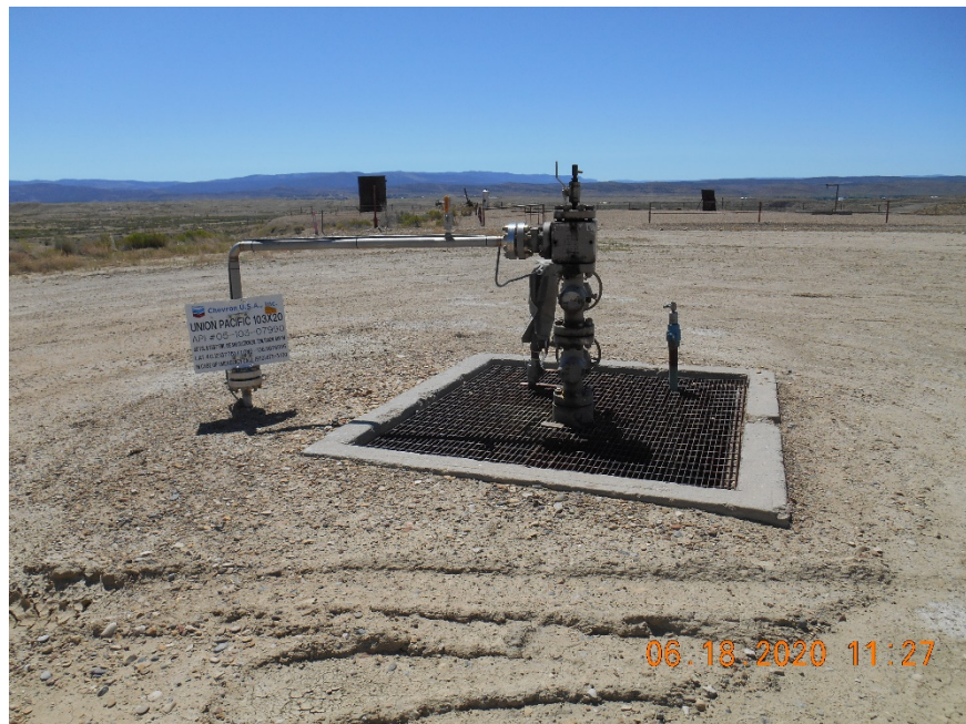
Injection wellhead
