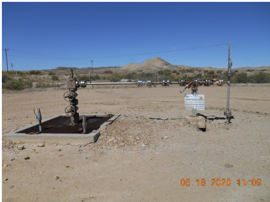
Injection wellhead
