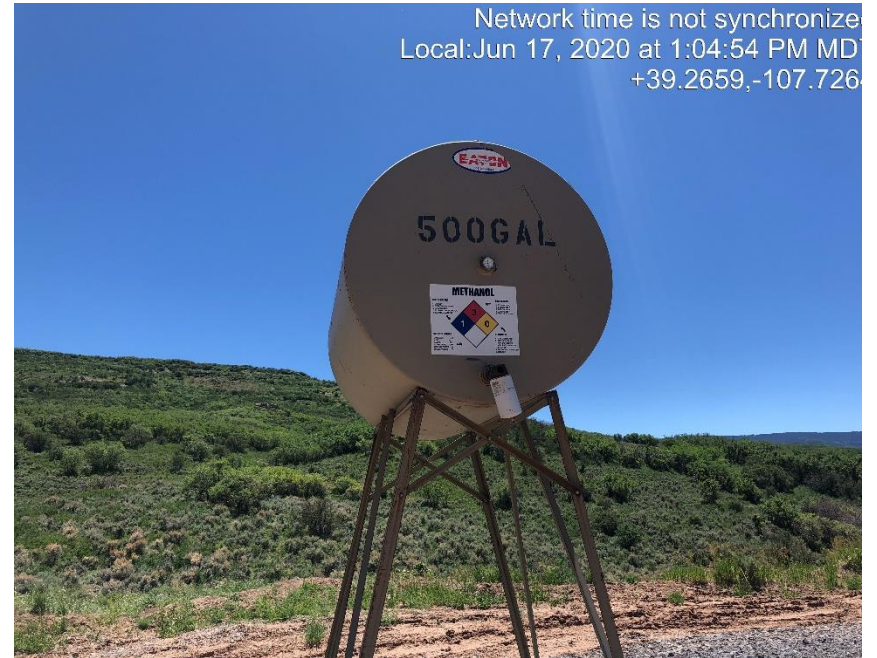
Photo #1383 500 gallon methanol tank missing operator name.
