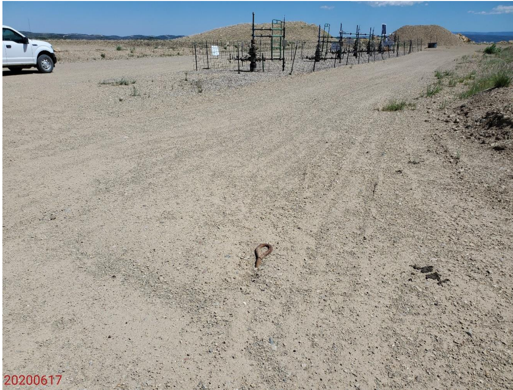
Photo 5: Photo shows example of anchors on the Location that are not marked pursuant to 1003 Rules.
