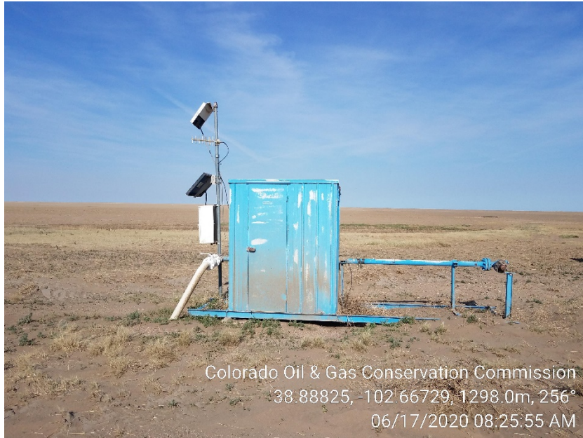
1. Meter Shed and pipeline risers
