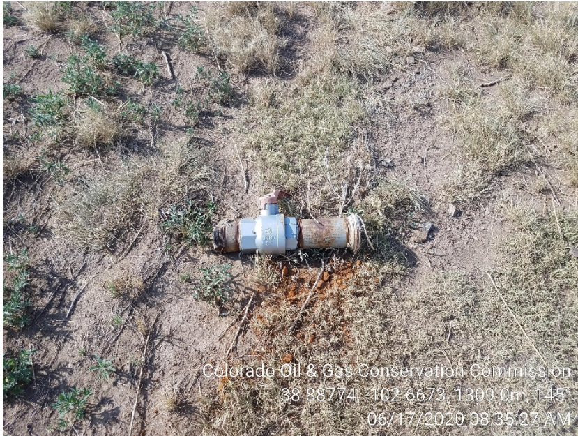
3. Valve broke off of tank
