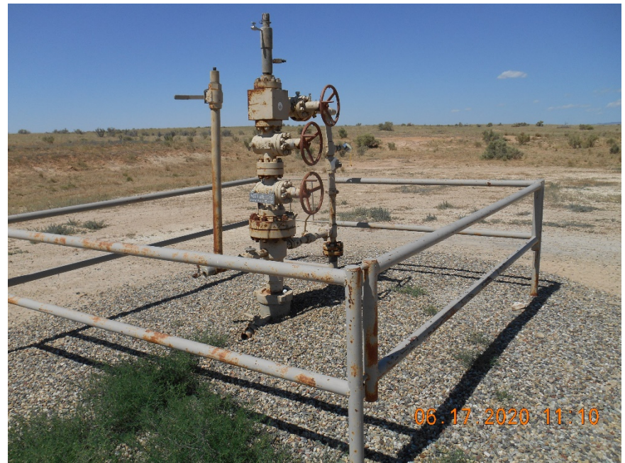
Wellhead Temporarily Abandoned
