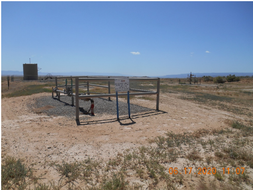
Location overview looking SE.
