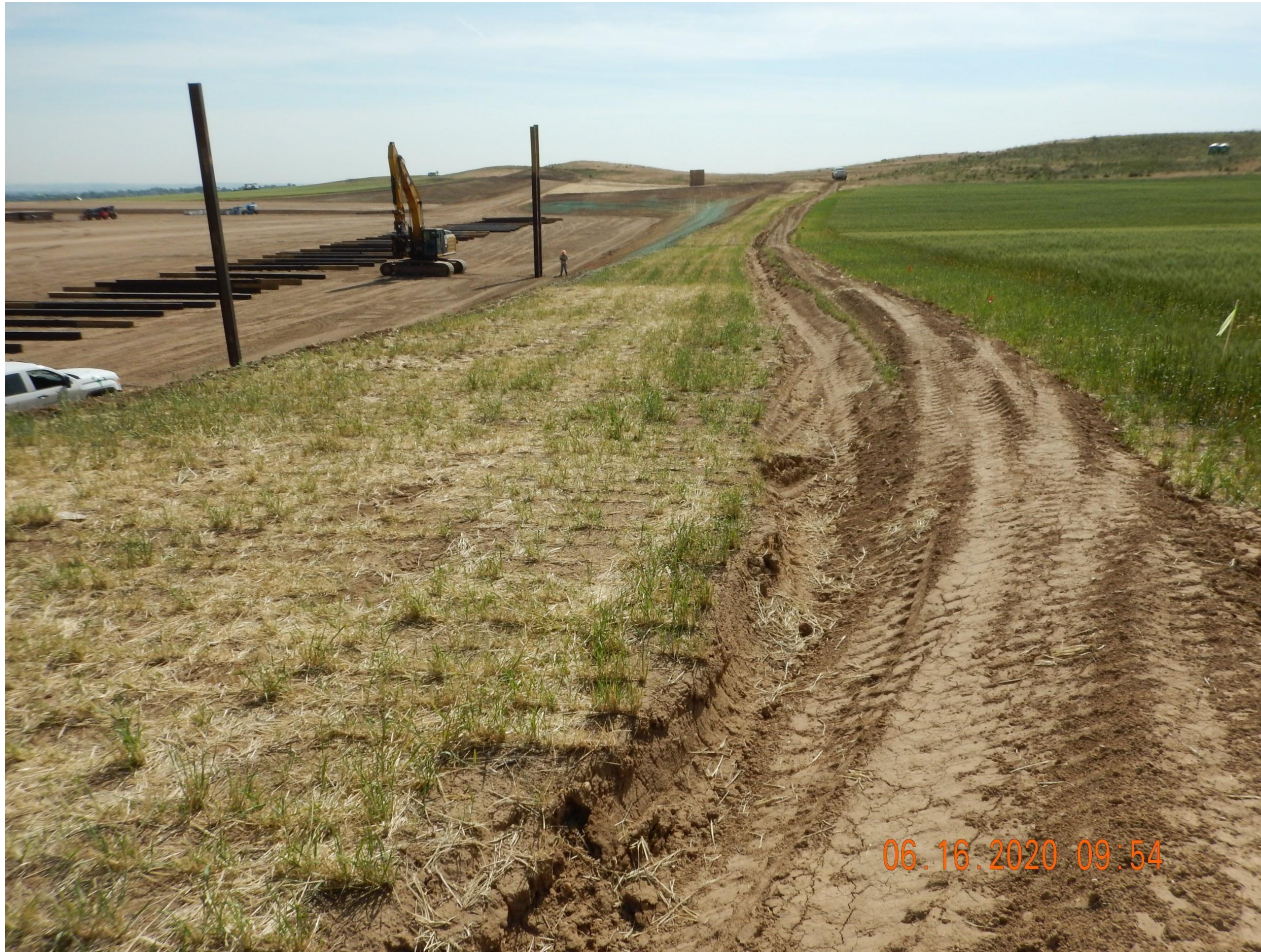
Photo 3. Photo taken from the southwestern location, facing East. See comments under Photo 2. Photo also illustrates the ditch and berm BMP that has been installed around the entire perimeter of location.
