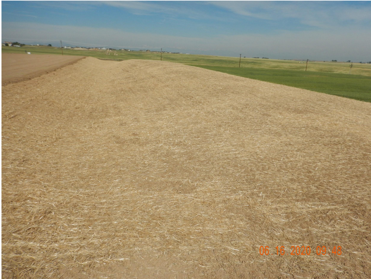
Photo 7. Photo taken from the northern location, facing West. Photo illustrates topsoil has been temporarily stabilized with equipment tracking and straw crimped mulch.
