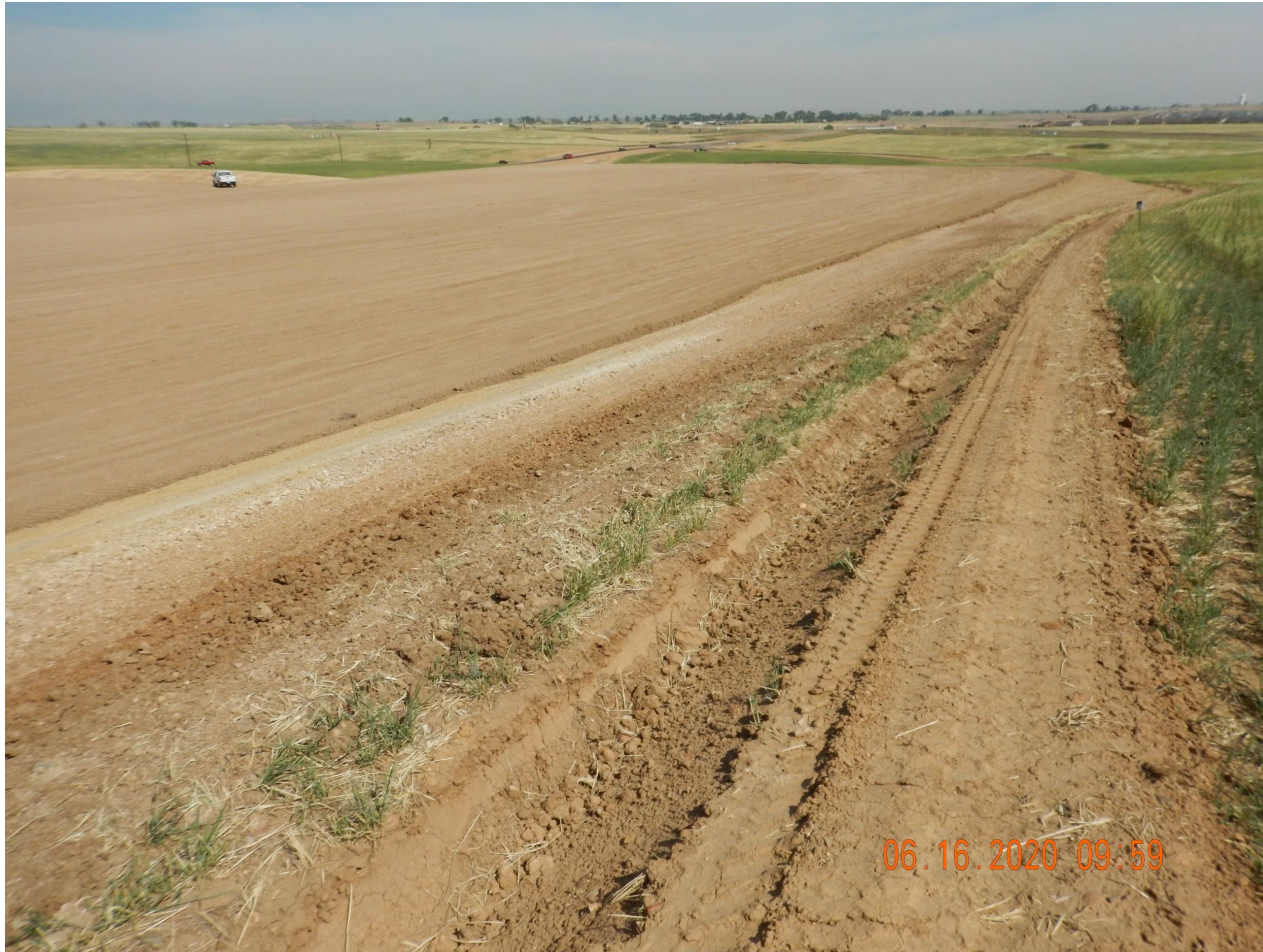
Photo 6. Photo taken from the southeastern location, facing Southwest. See comments under Photo 4. Photo also illustrates the ditch and berm BMP that has been installed around the entire perimeter of location.
