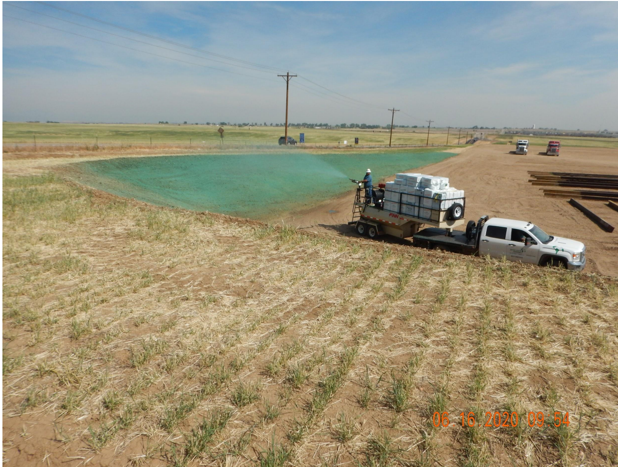
Photo 1. Photo taken from the southwestern location, facing North. Photo illustrates Operator is implementing temporary stabilization (i.e., hydromulch) along portions of the well pad cut slope .
