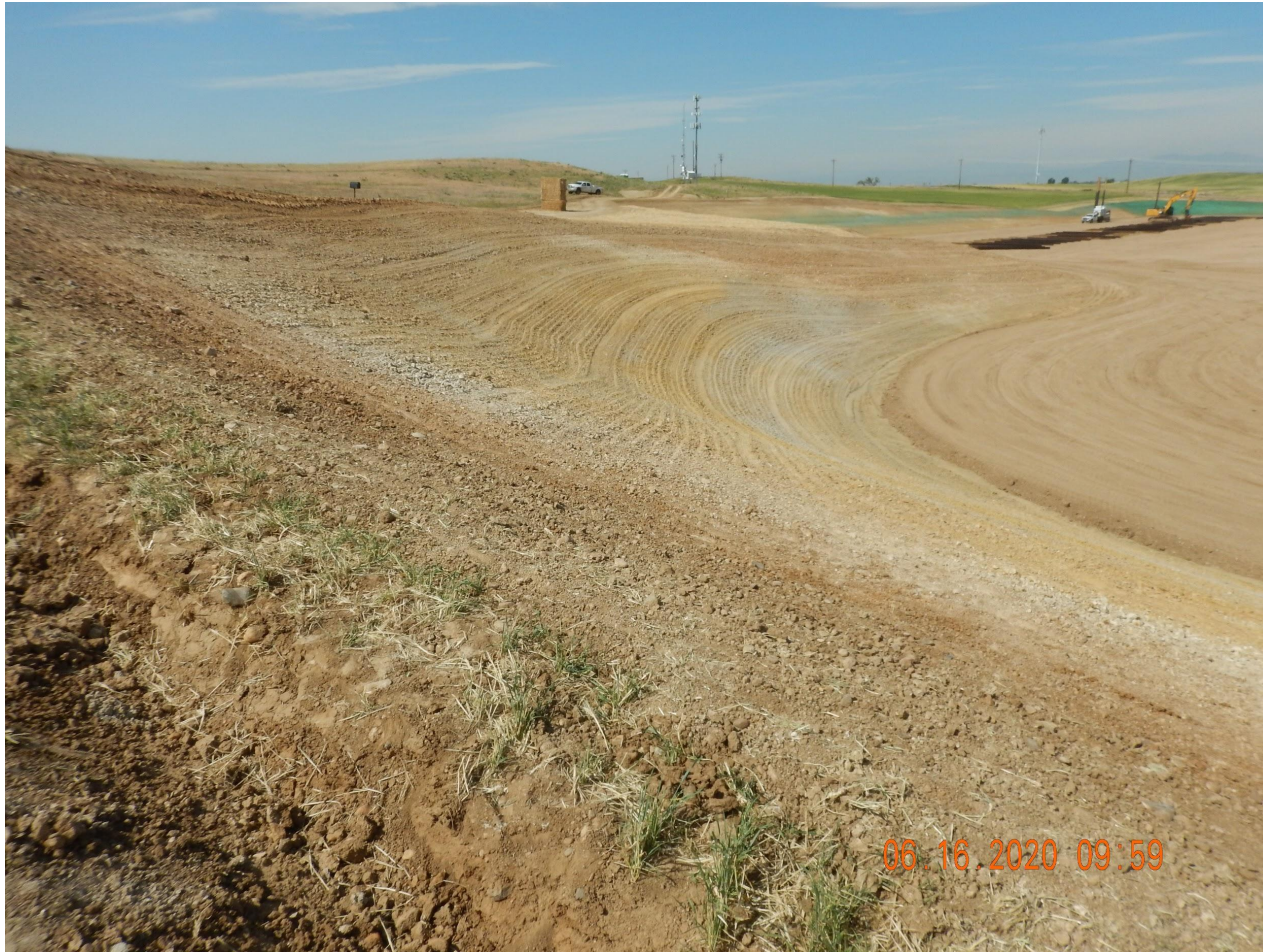
Photo 5. Photo taken from the southeastern location, facing Southwest. Photo illustrates Operator has temporarily stabilized the cut slope areas of the production facility.
