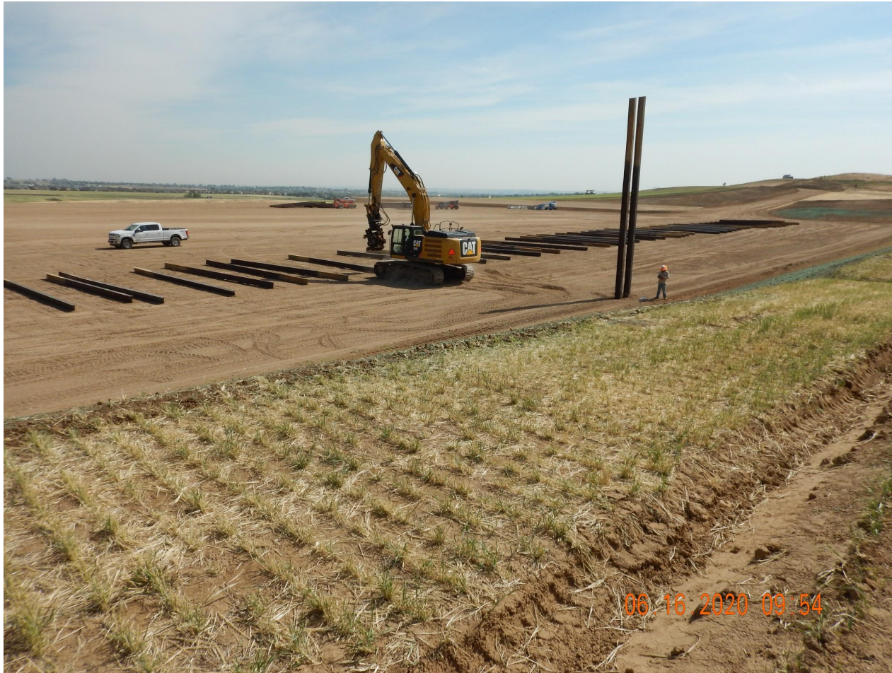
Photo 2. Photo taken from the southwestern location, facing Northeast. Photo illustrates Operator is in process of installing the sound wall along the southern well pad.
