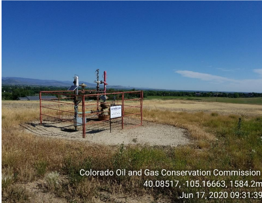
Photo 1 WH new well head sign well is shut in and LOTO
