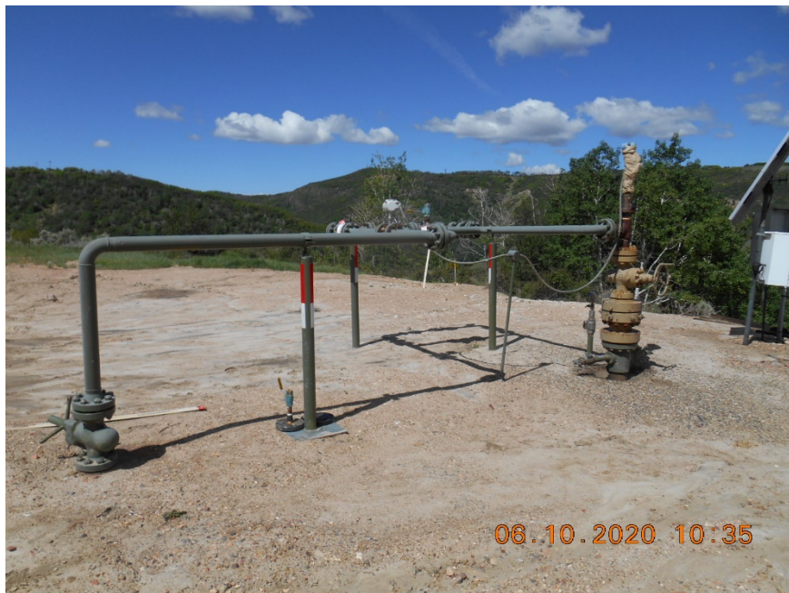
Injection wellhead
