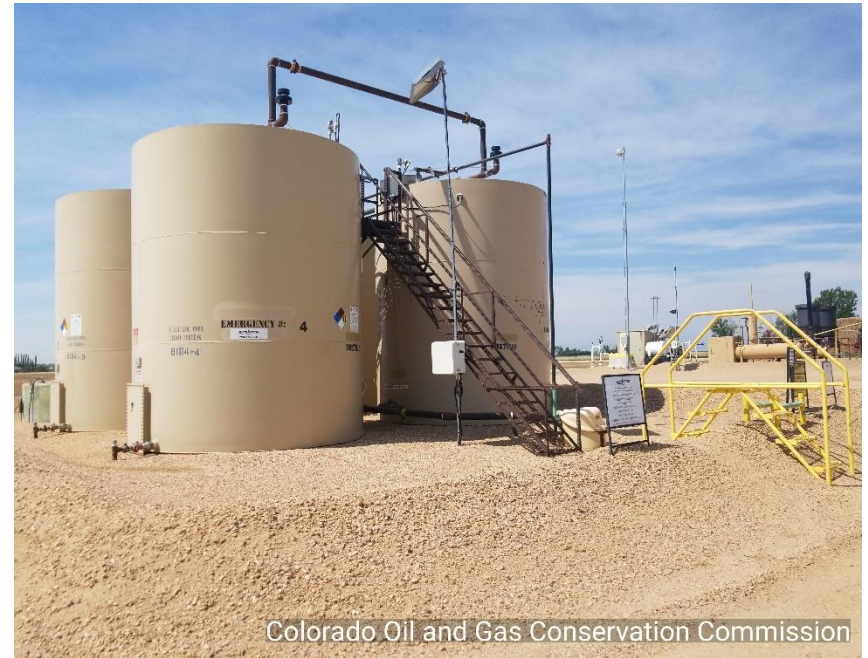
Photo 10: Tank Battery
