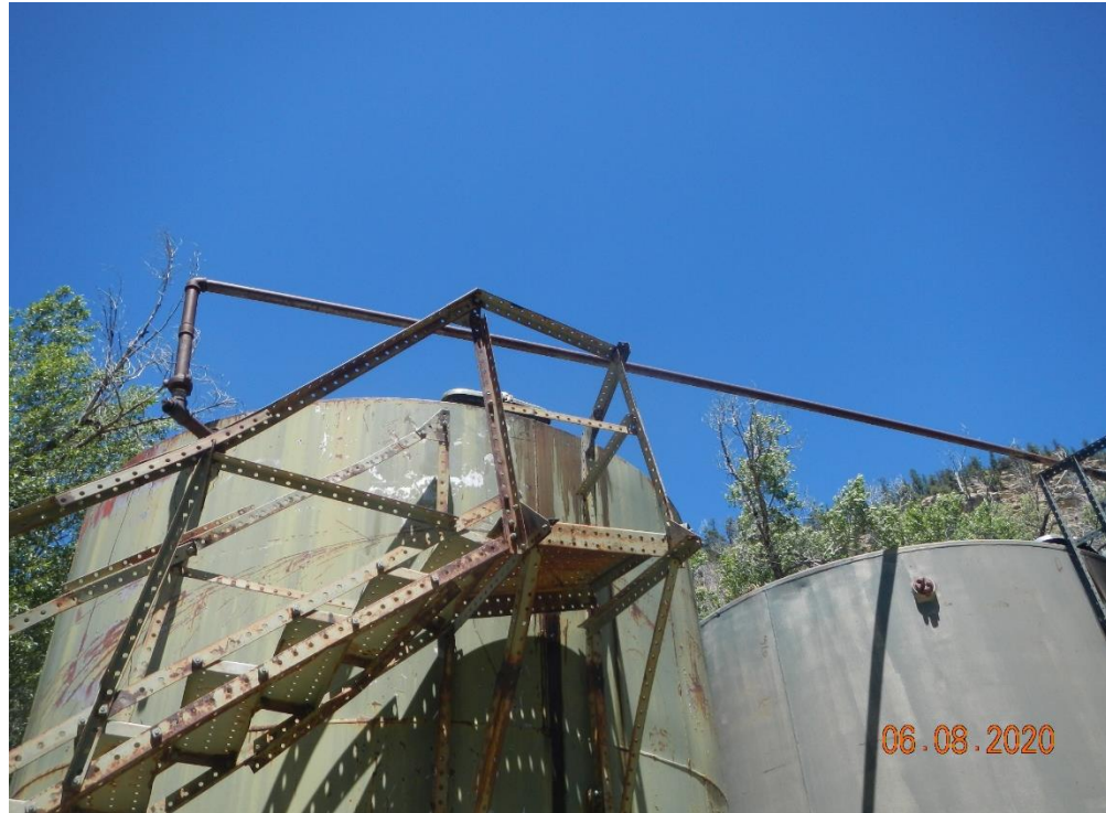
Crude oil running down side of tank
