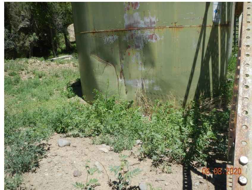
Weeds in berms, no anchoring in floodplain, south tank requiring paint
