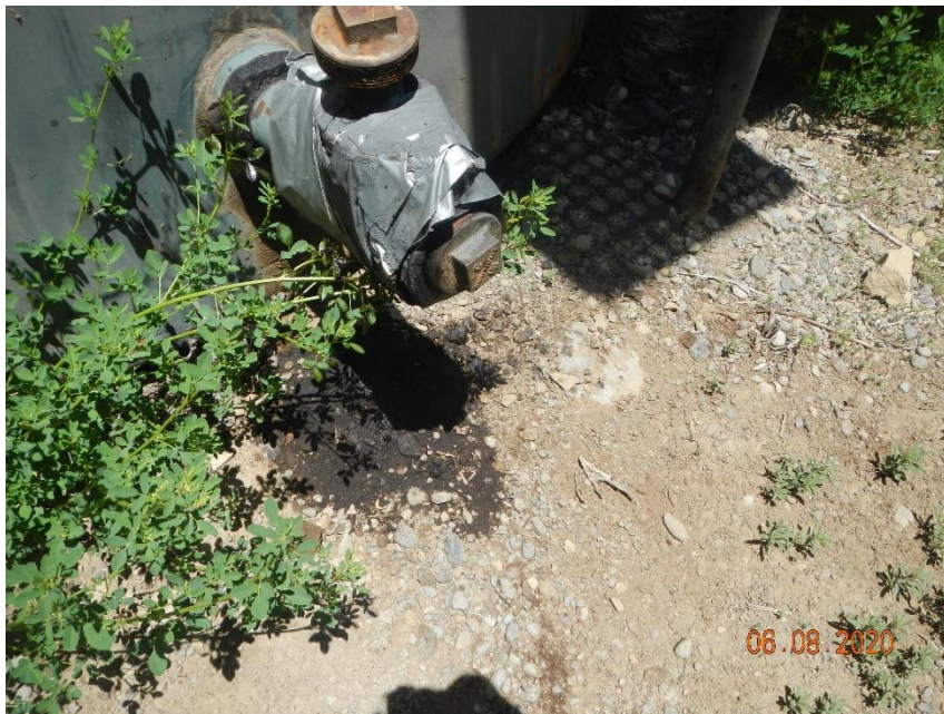
Oil stain, leaking valve north tank
