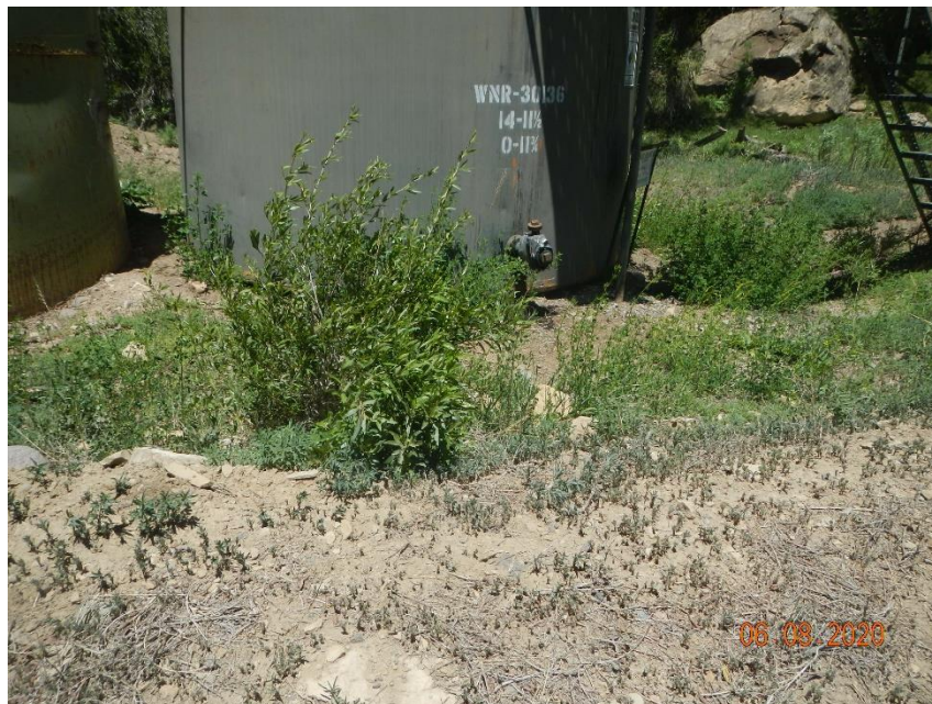
Weeds in berms, no anchoring or steel ring in floodplain
