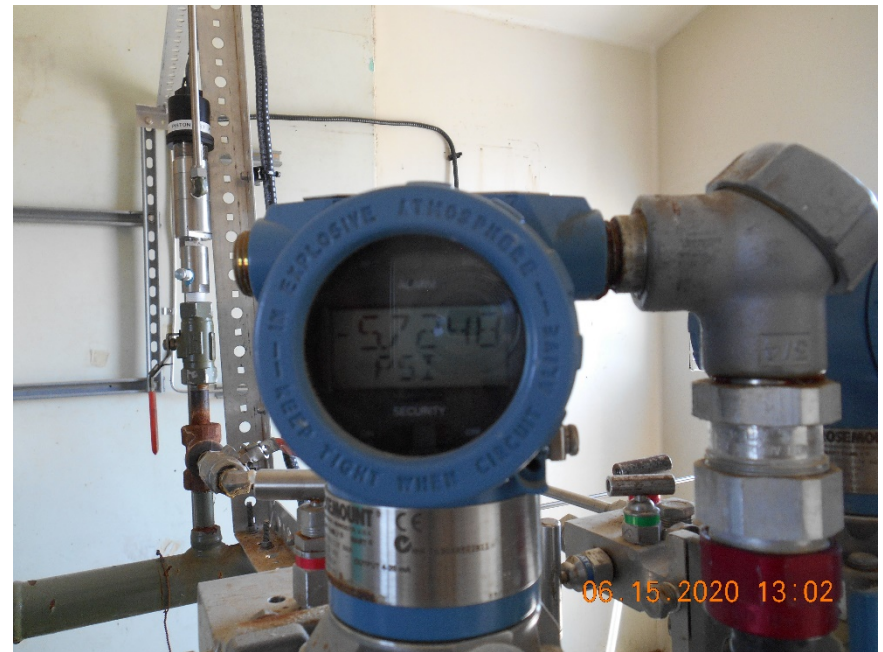
Injection well tubing gauge.
