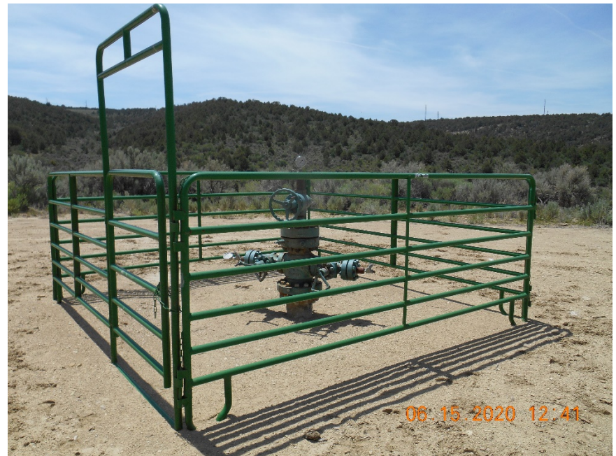
Injection Wellhead Temporarily Abandoned
