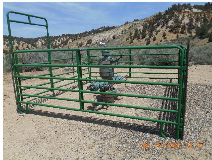
Injection Wellhead Temporarily Abandoned
