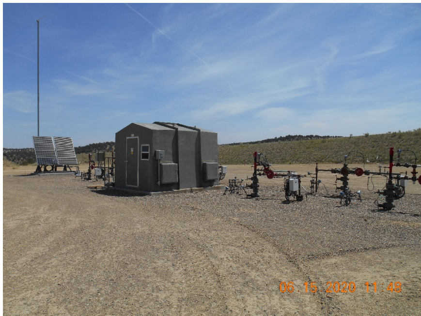
Injection well housing
