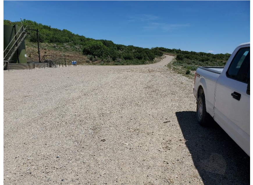
Photo 4: See comments under photo 1.
