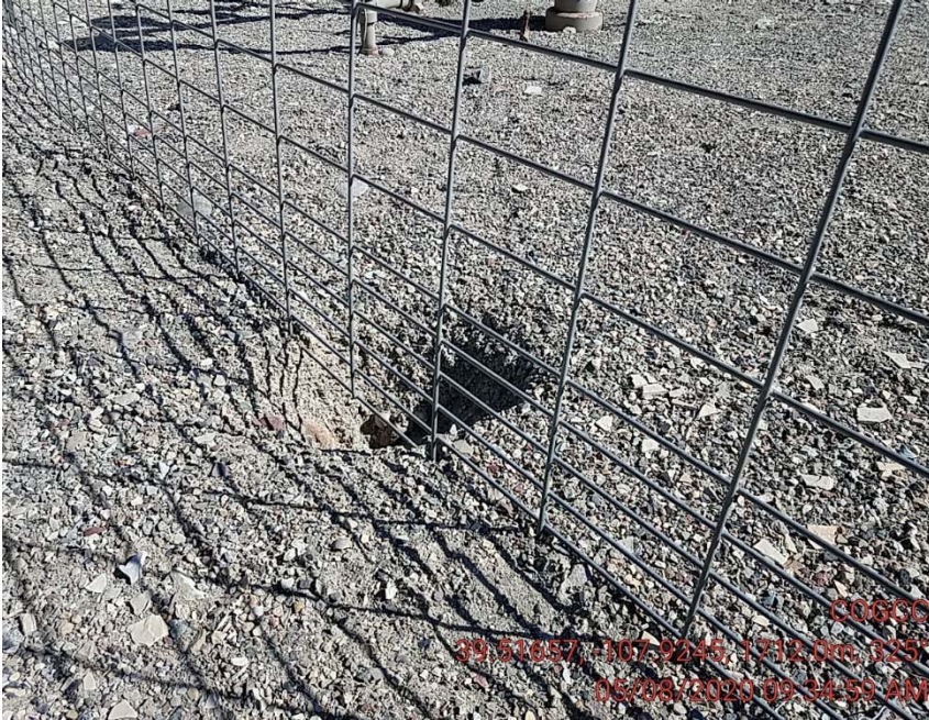
Previous inspection photo
