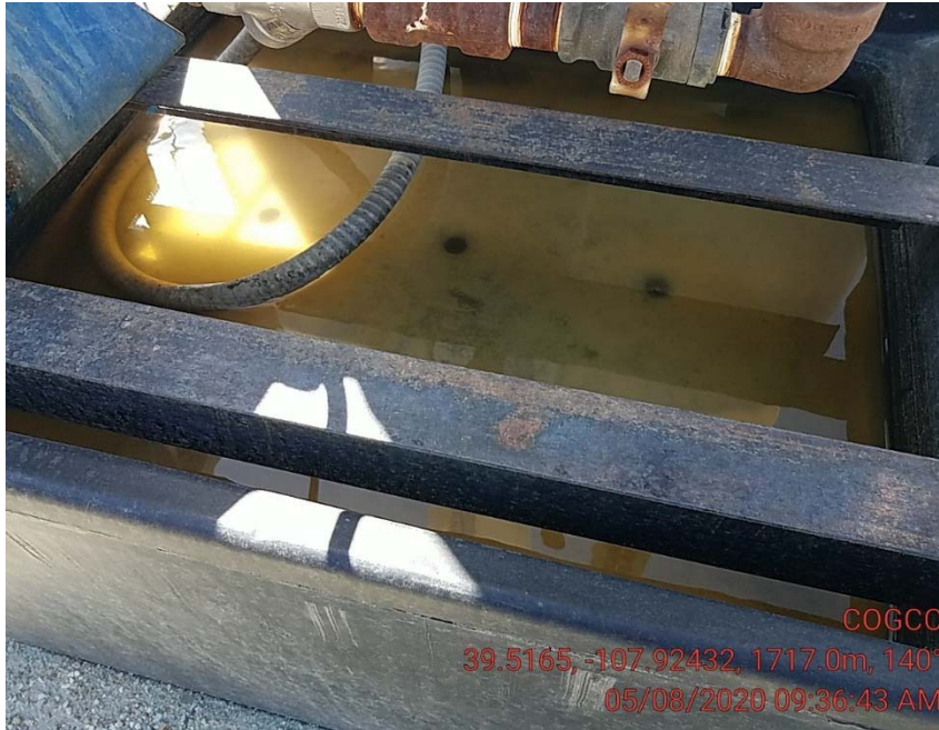
Previous inspection photo
