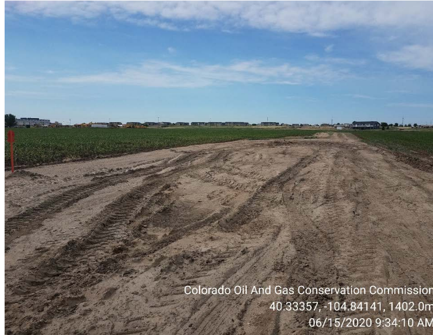
Production facility on 6/15/2020
