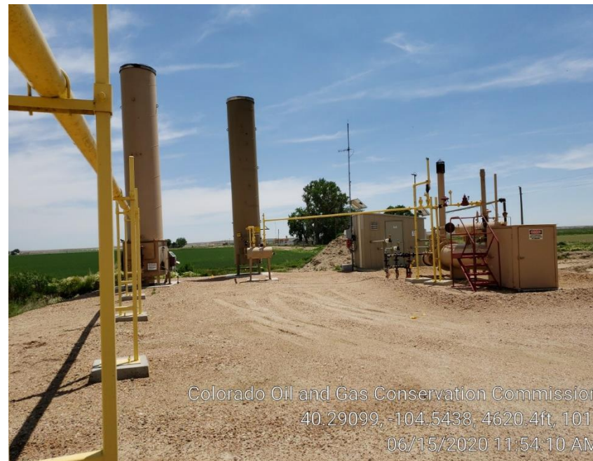
Photo #4 Separator, ECDs & Meter Run
