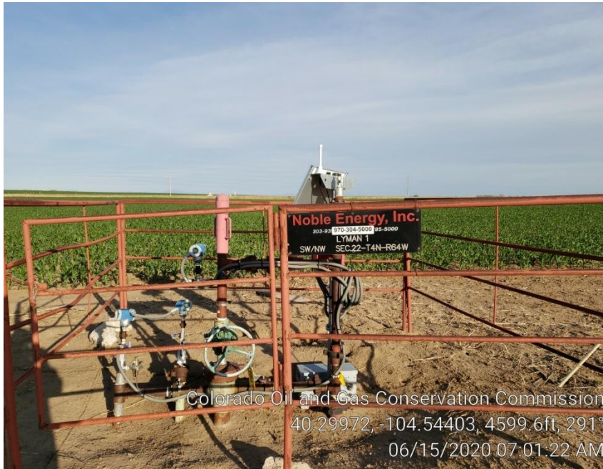
Photo #1 Well & Sign
