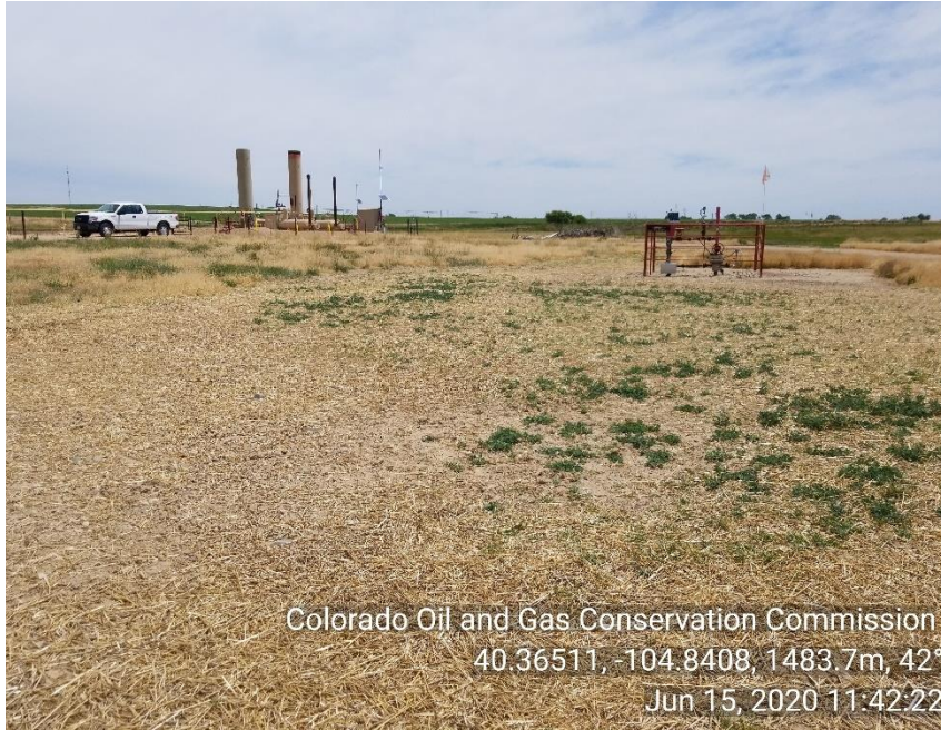
Photo 5: Location of PA wellheads
