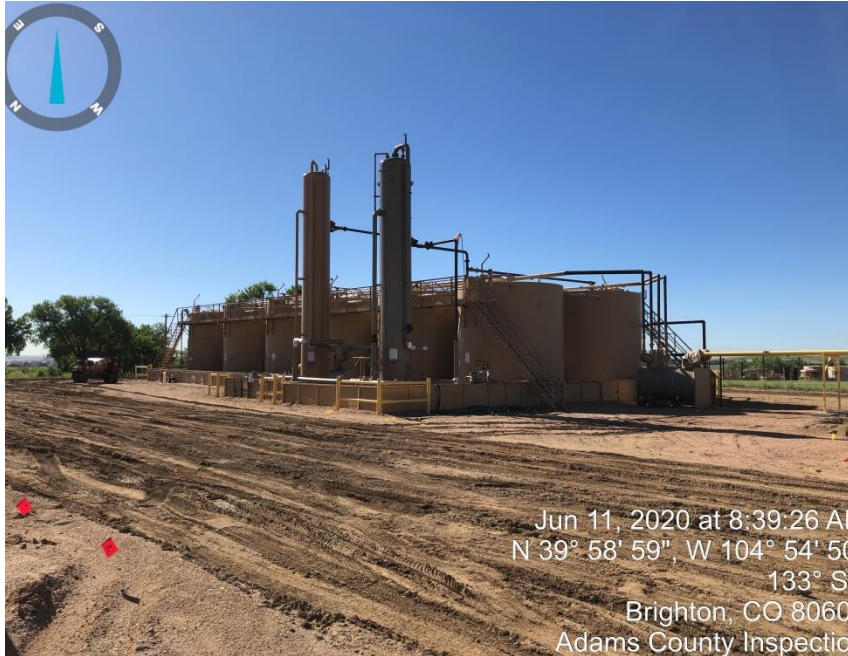
Photo#1 Tank battery
