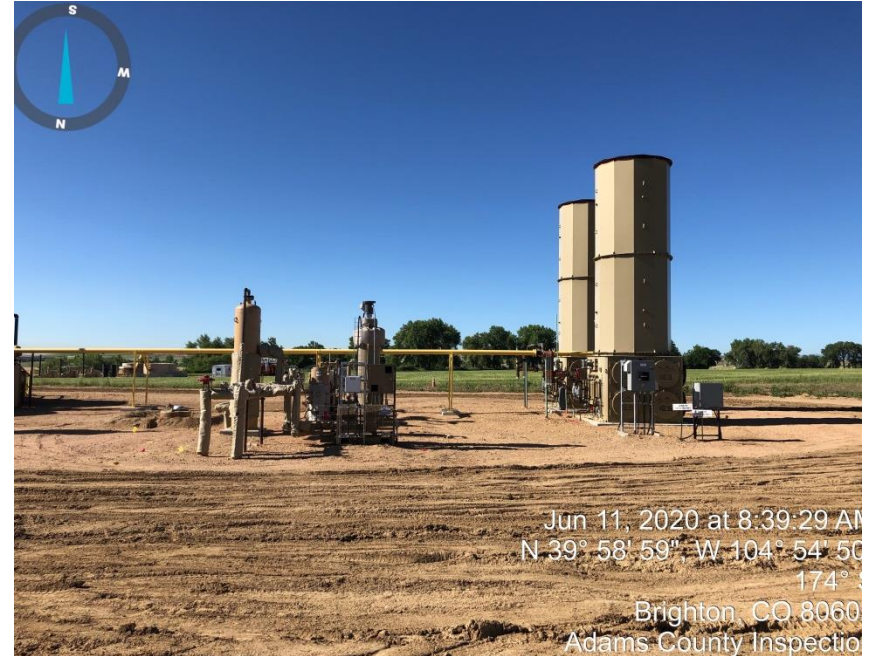
Photo#2 ECDs/ECO Unit Recovery Unit
