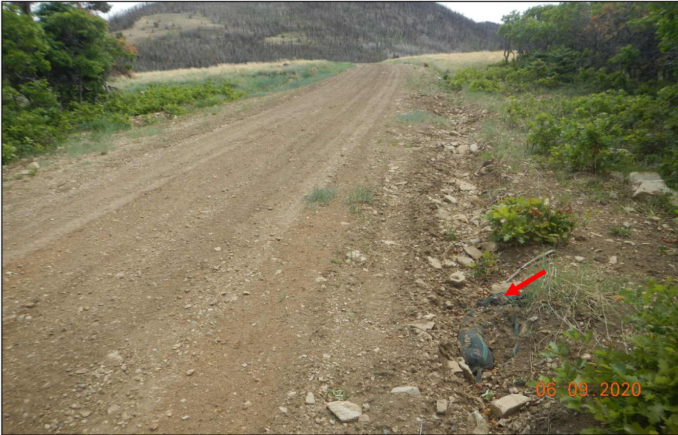
Photo 1. Facing south ascending the hill toward the location. The BMP's along the side of the road are not maintained. Red arrow points to rock wattle.
