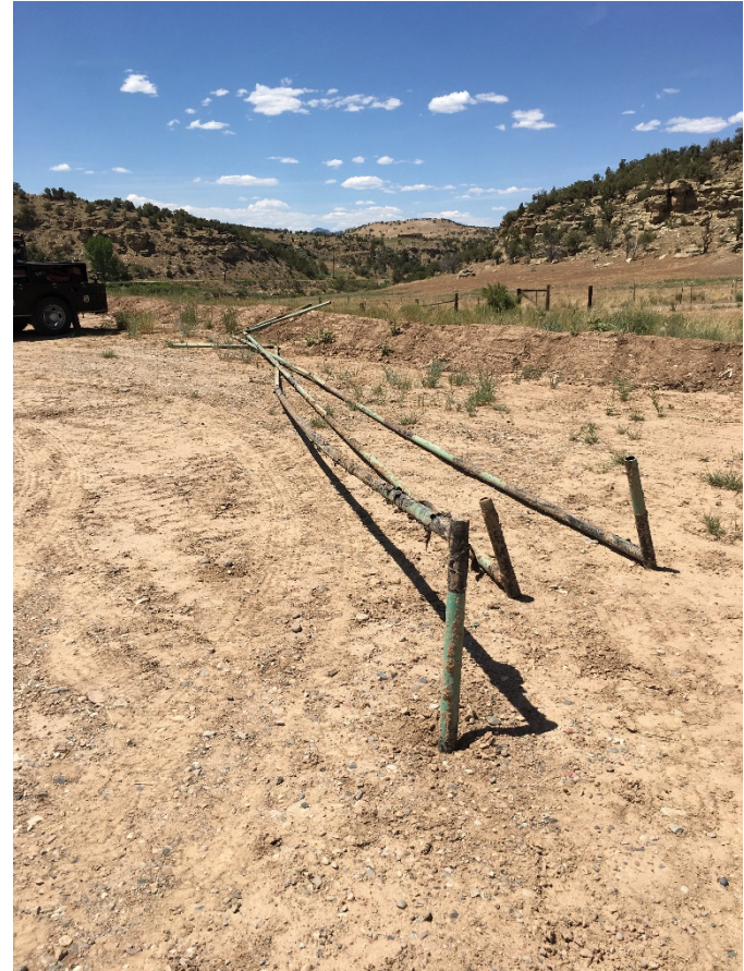
Flowlines removed and taken out of service, Flowlines from separator to tank battery
