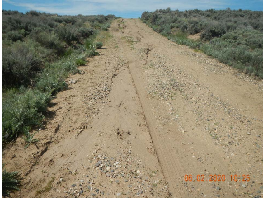
Photo 3. Example of erosion rills on access road.
