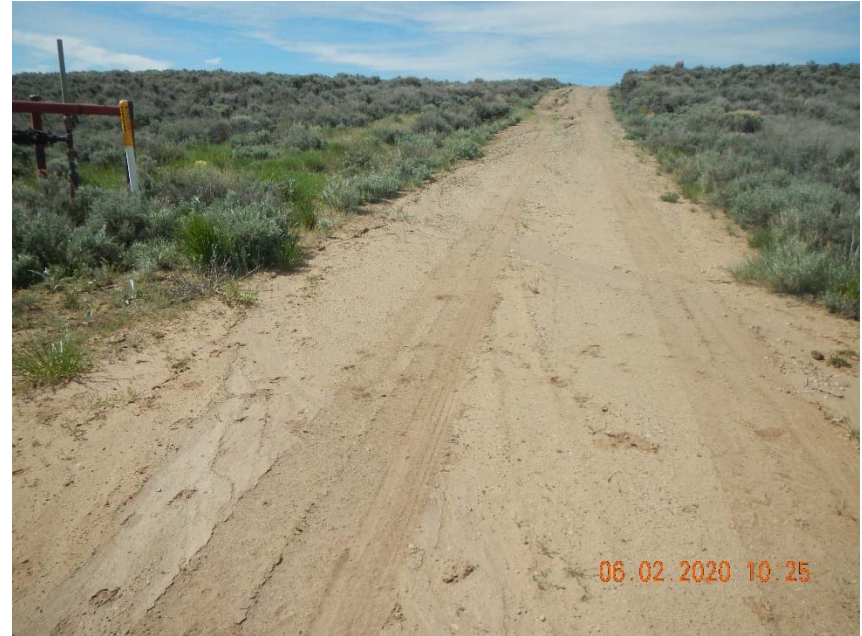
Photo 2. Example of erosion rills on access road.
