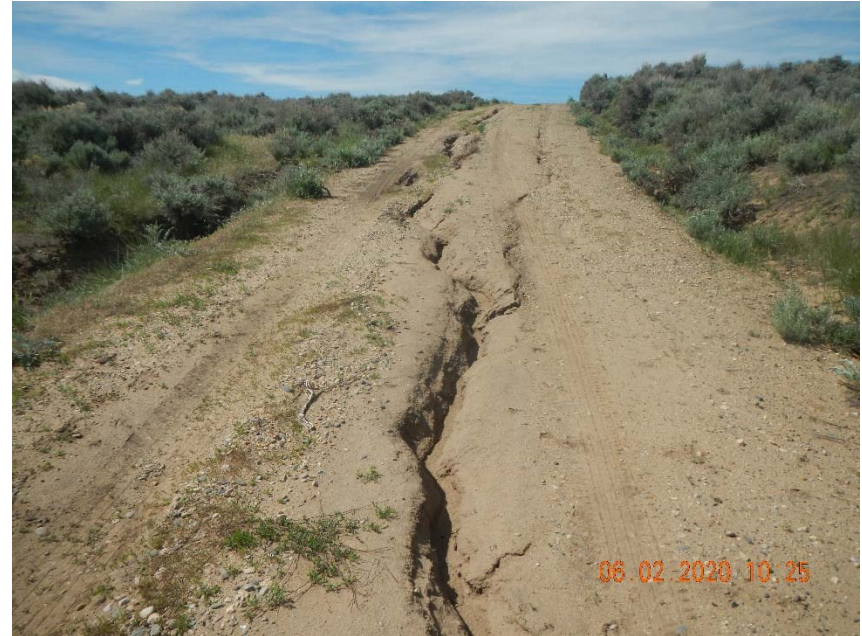
Photo 4. Example of erosion rills on access road.
