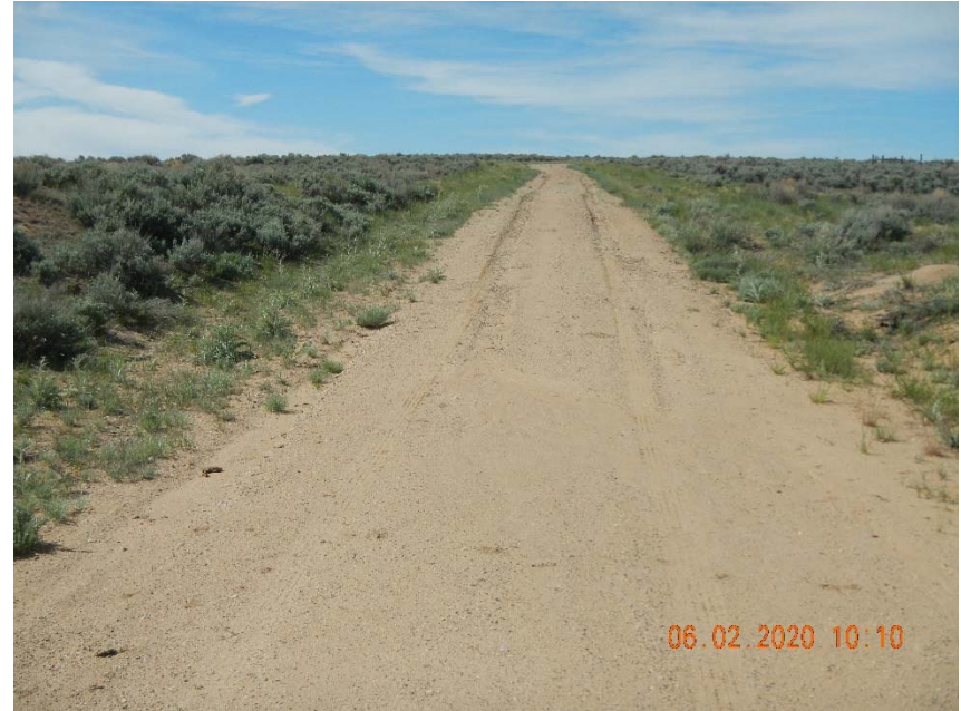
Photo 3. Example of erosion rills on access road.
