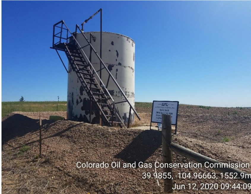
Photo 3 tank paint in disrepair
