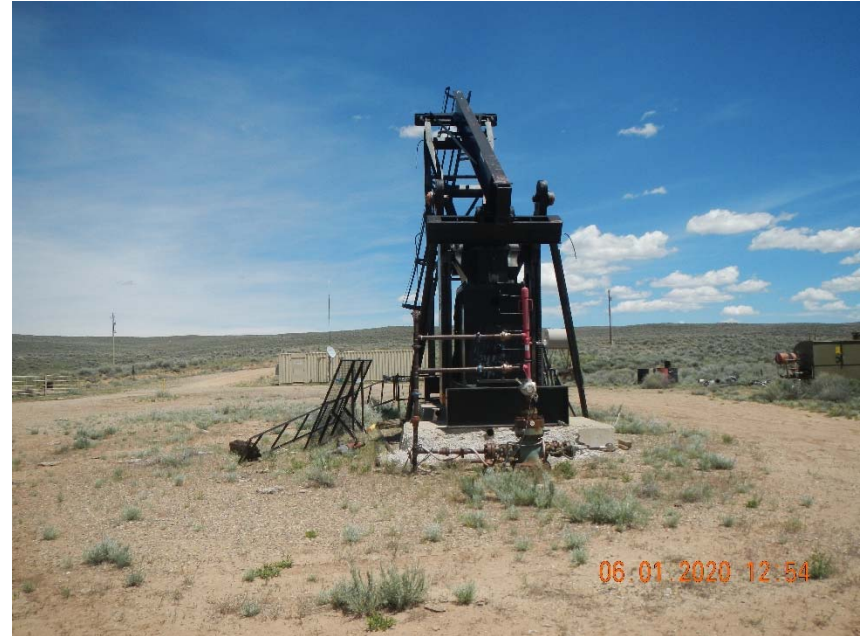
Photo 10. No wellhead sign, equipment stored on location.
