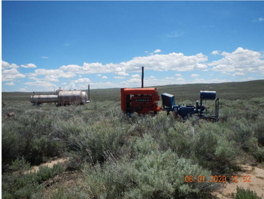
Photo 7. Example of debris, trash, equipment on location.
