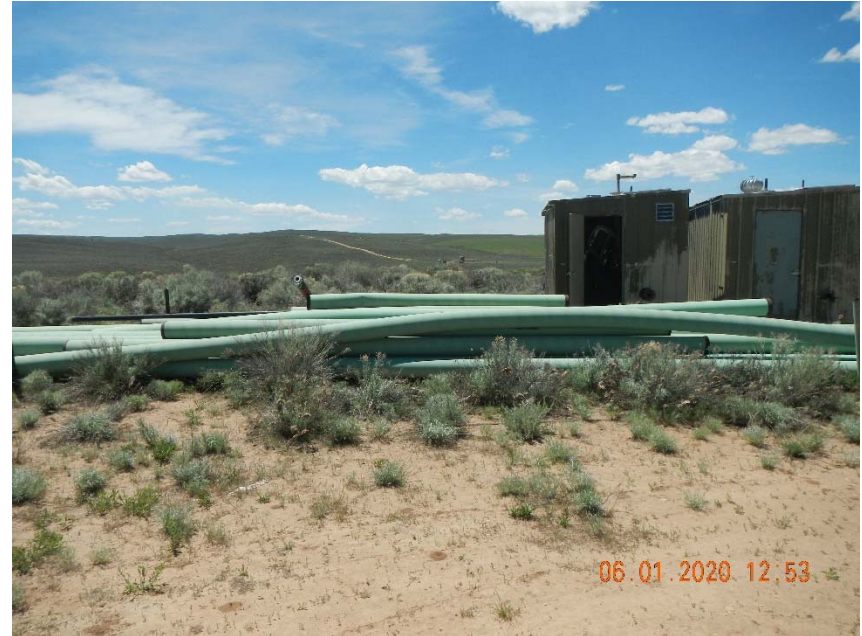
Photo 8. Example of debris, trash, equipment stored on location.
