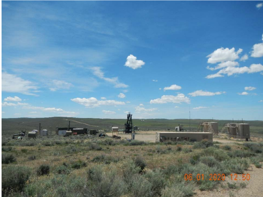
Photo 1. Overview of location taken facing southwest.
