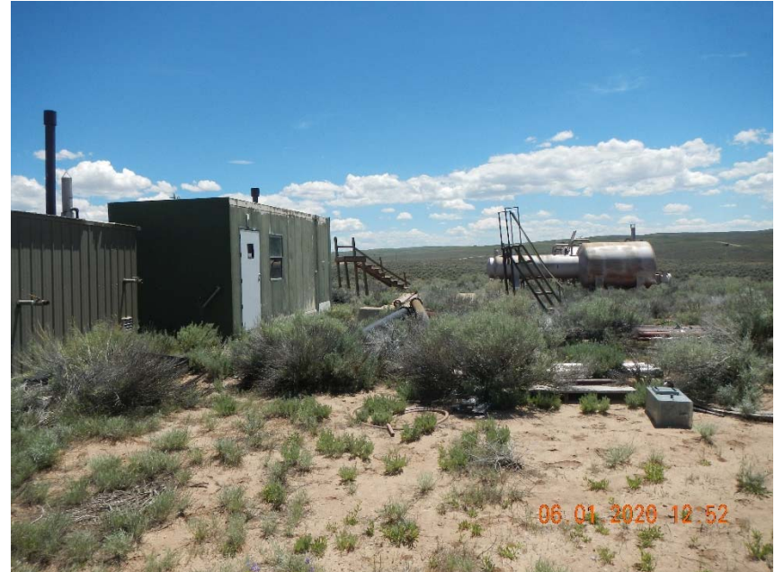
Photo 6. Example of debris, trash, equipment stored on location.
