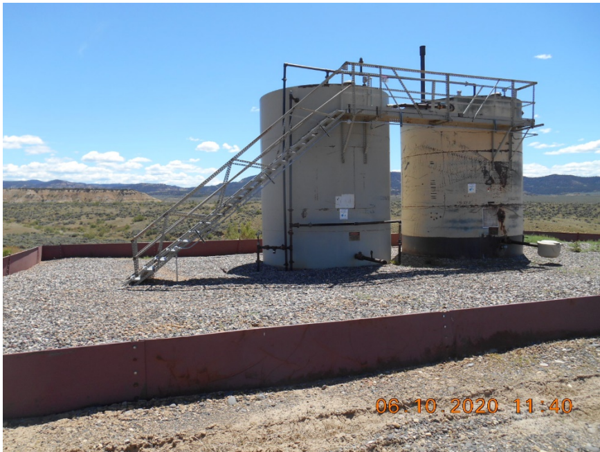
Production tank battery
