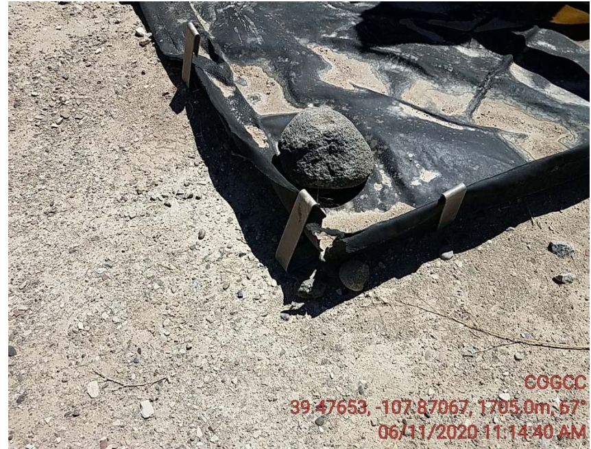
Secondary containment under pump
