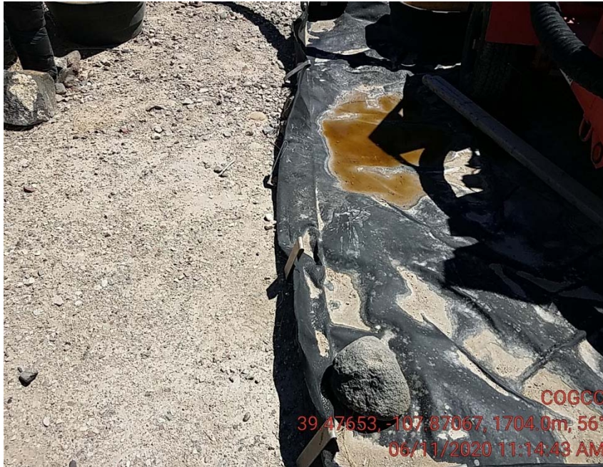
Secondary containment under pump
