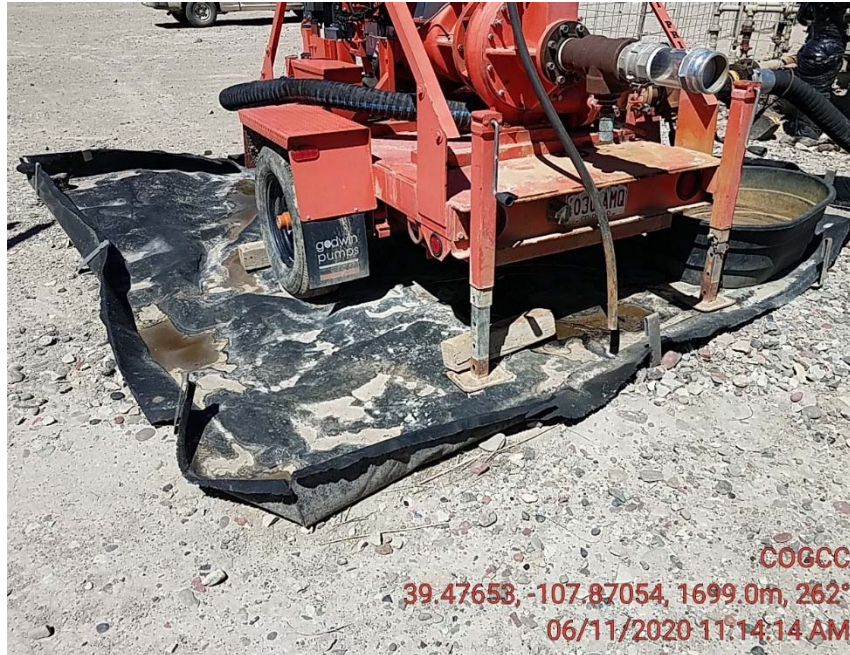
Secondary containment under pump
