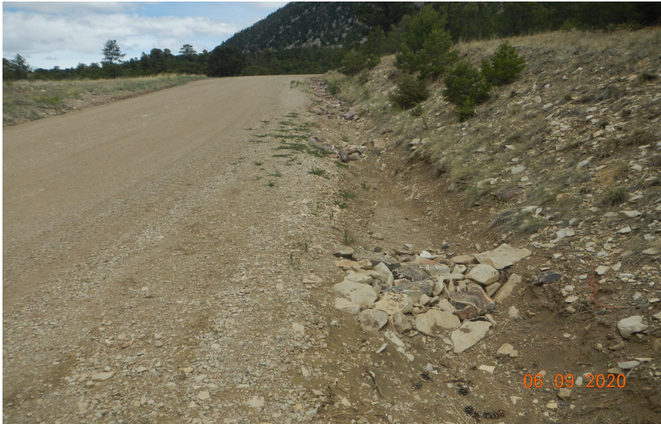
Photo 1. Facing northeast along the main road. Rock checkdamns have been repaired since previous inspection. Lat/Long:37.69860,-105.21673
