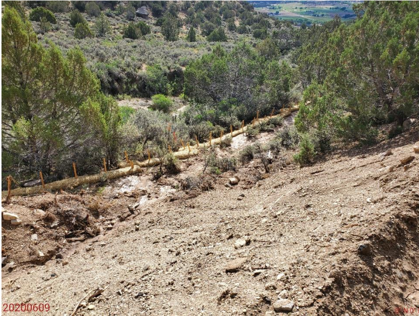
Photo 21: Photo taken from the access road, facing southwest. Photo shows areas where sediment deposition has begun filling the wattle BMPs. Advised maintenance prior to BMP failure.
