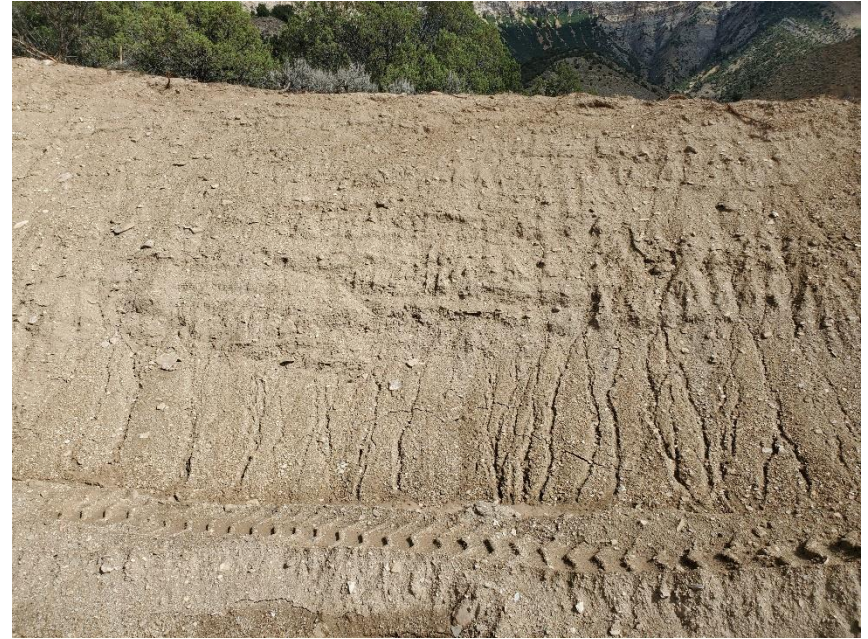
Photo 14: Photo taken from the north end of the Location, facing north. Photo shows soils on cut slopes. BMPs to stabilize and protect slopes appear insufficient or missing; Erosion degradation evident.
