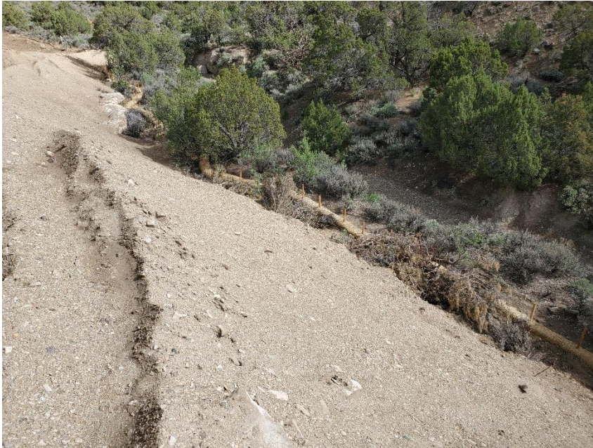
Photo 17: Photo taken from the east end of the Location, facing north. Photo shows soils on the fill slopes. BMPs to stabilize and protect slopes appear insufficient or missing
