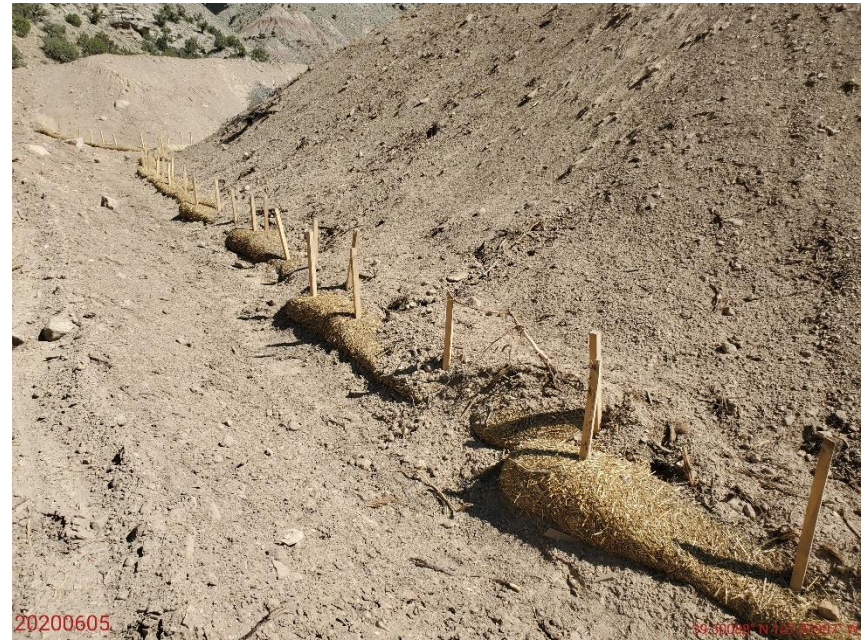
Photo 6: Photo taken from the soil stockpile. Photo shows Operator has installed hay bale and wattle BMPs at the toe of the soil stockpile. BMPs have filled with sediment and are no longer in proper functioning condition. BMPs used in conjunction with hay bale/wattles are missing, or insufficient to stabilize the soils of the stockpile.
