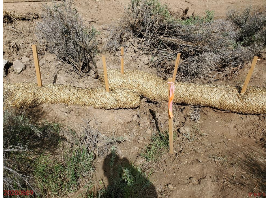
Photo 20: Continued from photo 18. Photo shows point where stormwater discharges. Photo shows that the Wattle BMP is not in proper functioning condition; Stormwater appears to have cut under the wattle resulting and erosion degradation and off-site sediment discharge.
