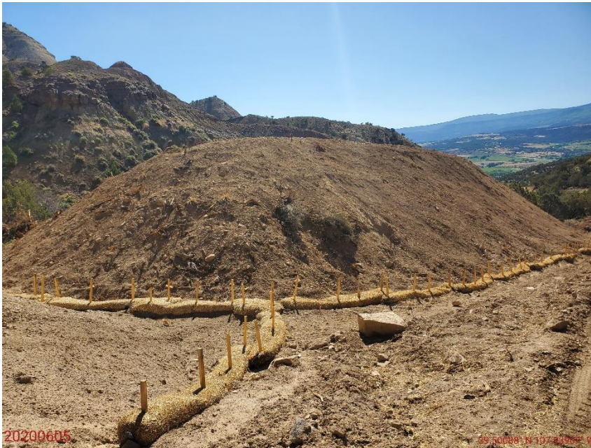
Photo 5: Photo taken from the south end of the Location, facing south. Photo shows soil stockpile on the Location; No other soil stockpiles appear to have been constructed. Photo also shows Operator has installed hay bale and wattle BMPs at the toe of the soil stockpile. Additional BMPs to stabilize the soils of the stockpile appear missing, or insufficient.
