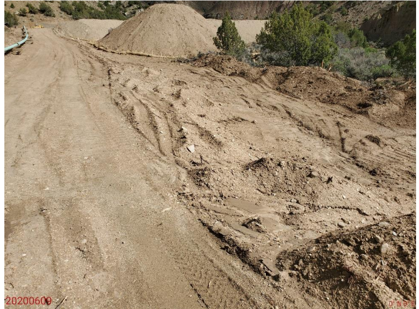
Photo 18: Photo taken from the access road, south of the Location. Photo shows area where stormwater runoff from the pad and access road concentrates and discharges.
