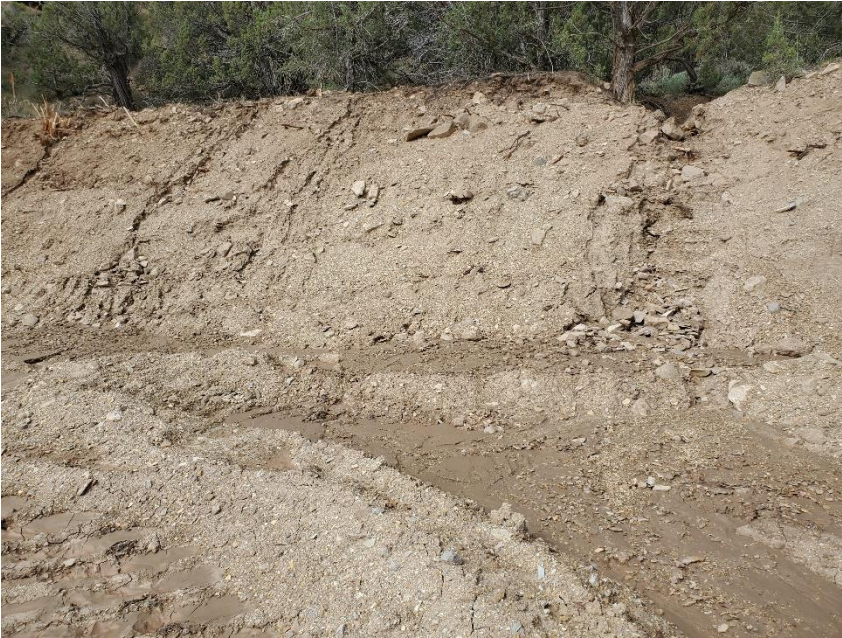
Photo 15: Photo taken from the west end o the Location, facing west. Photo shows soils on cut slopes. BMPs to stabilize and protect slopes appear insufficient or missing; Erosion degradation evident.
