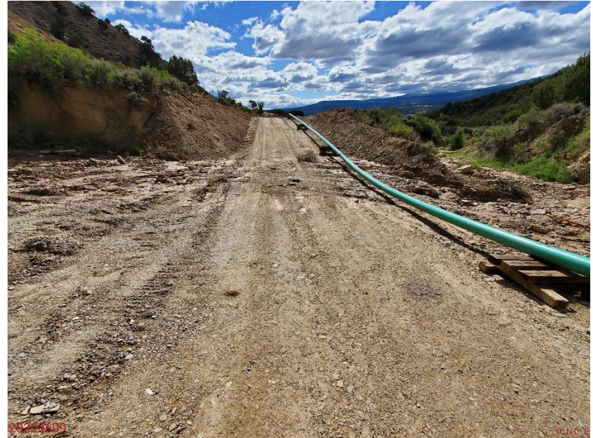
Photo 22: Photo taken from where access road crosses drainage. Photo shows BMPs to stabilize access road appear missing or insufficient.
