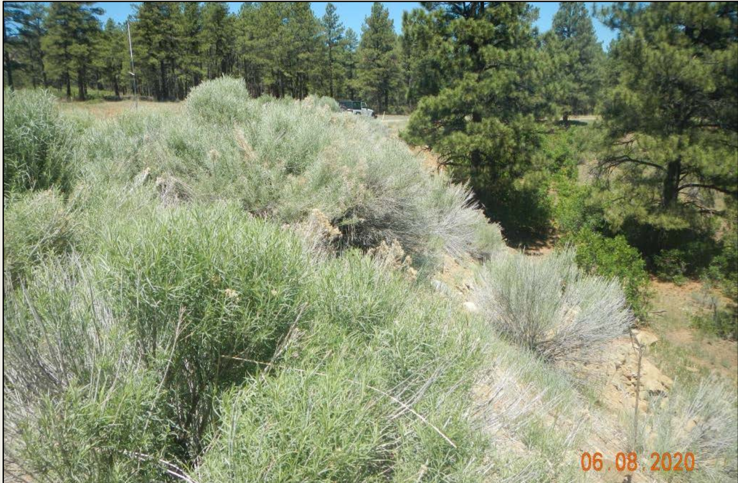
Photo 2. View of the eastern fill slope from the southeastern corner facing northward. Revegetation is progressing with western wheatgrass and rubber rabbitbrush.
