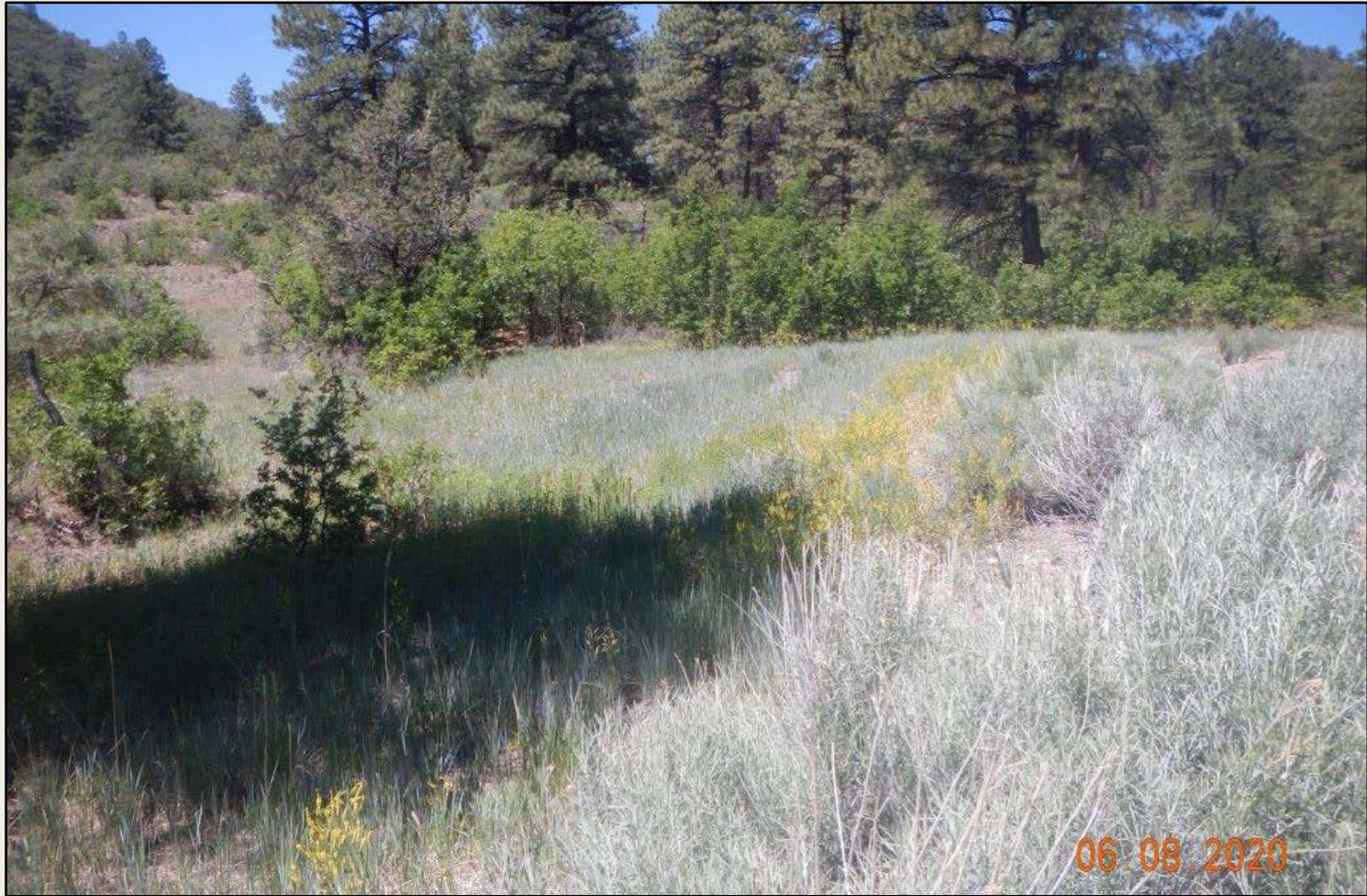
Photo 3. View of the eastern fill slope from the southeastern corner facing northward. Revegetation is progressing with western wheatgrass and rubber rabbitbrush.
