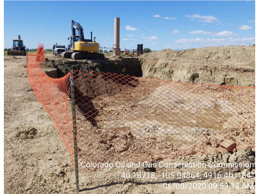
Photo 6 – Southern sidewall of excavation; stained soil observed in sidewalls under excavator. Orange safety fencing around inactive excavation extents.
