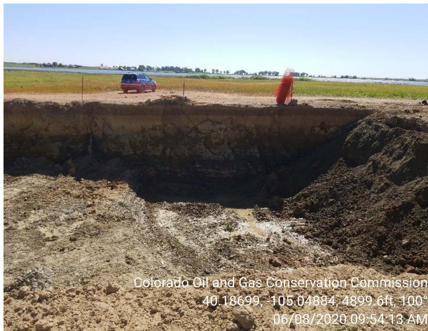
Photo 7 – Eastern sidewall of excavation. Goundwater seeping in through floor of excavation.
