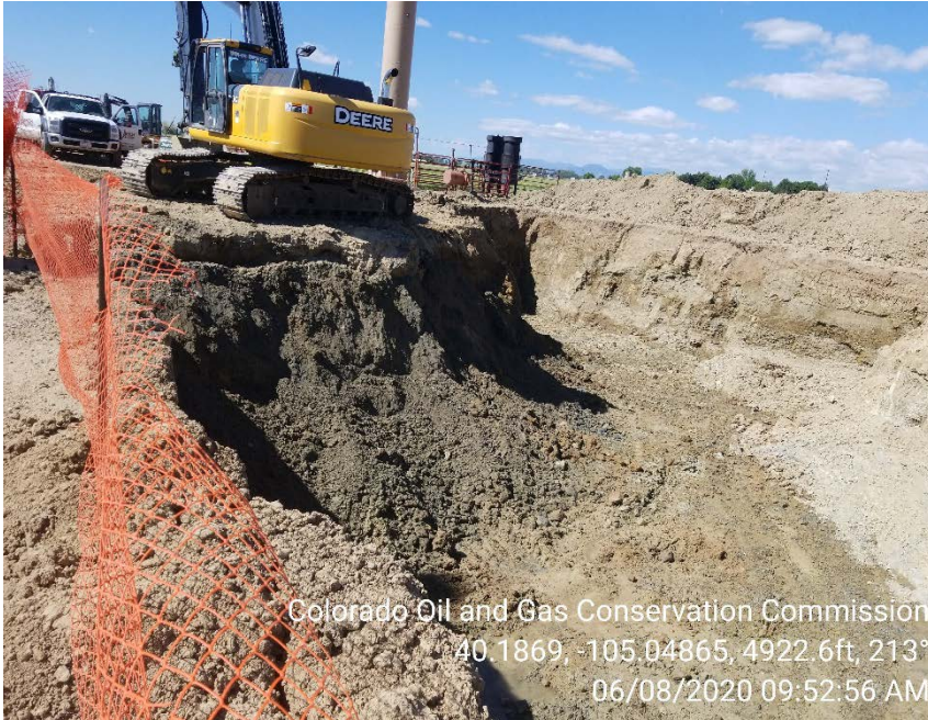
Photo 3 – Stained soil observed in southeast portion of the excavation.
