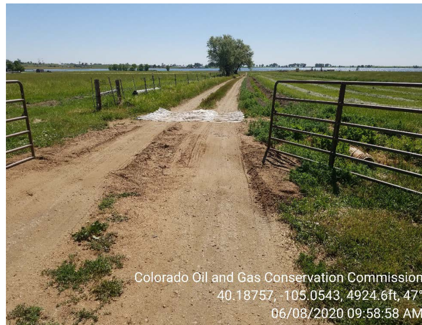
Photo 8 – Tracking pad at beginning of access road.
