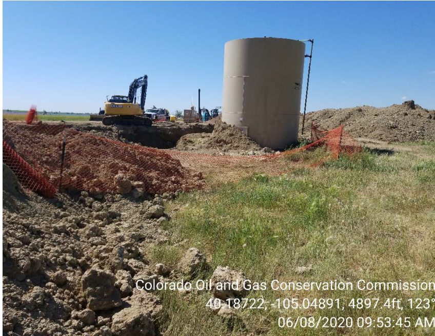
Photo 5 – Orange safety fencing around inactive parts of the excavation.
