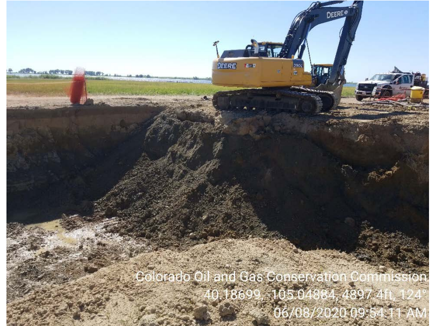
Photo 4 – Stained soil observed in sidewalls under excavator (southeast portion of the excavation).
