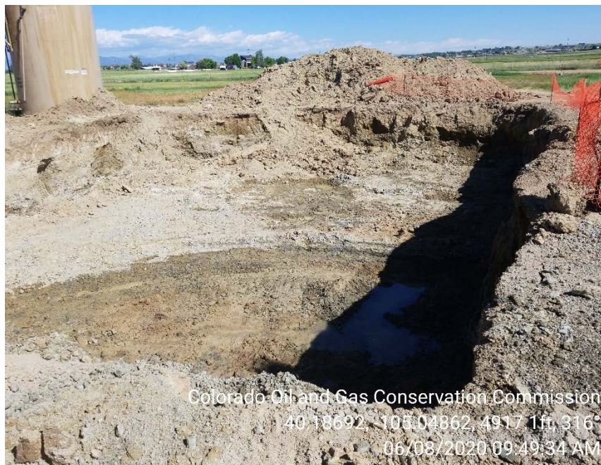
Photo 1 –Northern sidewall of excavation. Groundwater seeping in through deepest portions of the excavation
