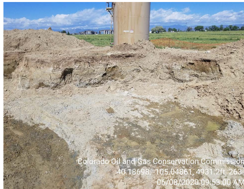
Photo 2 – Western sidewall of excavation. Groundwater seeping in through deepest portions of the excavation
