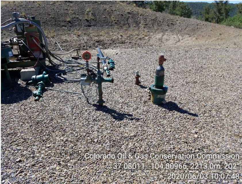
PHOTO 5: UNUSED EQUIPMENT (TWO UNUSED 2" RISERS & ONE 1" RISER). REMOVE UNUSED EQUIPMENT COMPLY WITH NTO AND RULE 603.F. CA DATE 9-3-20.
