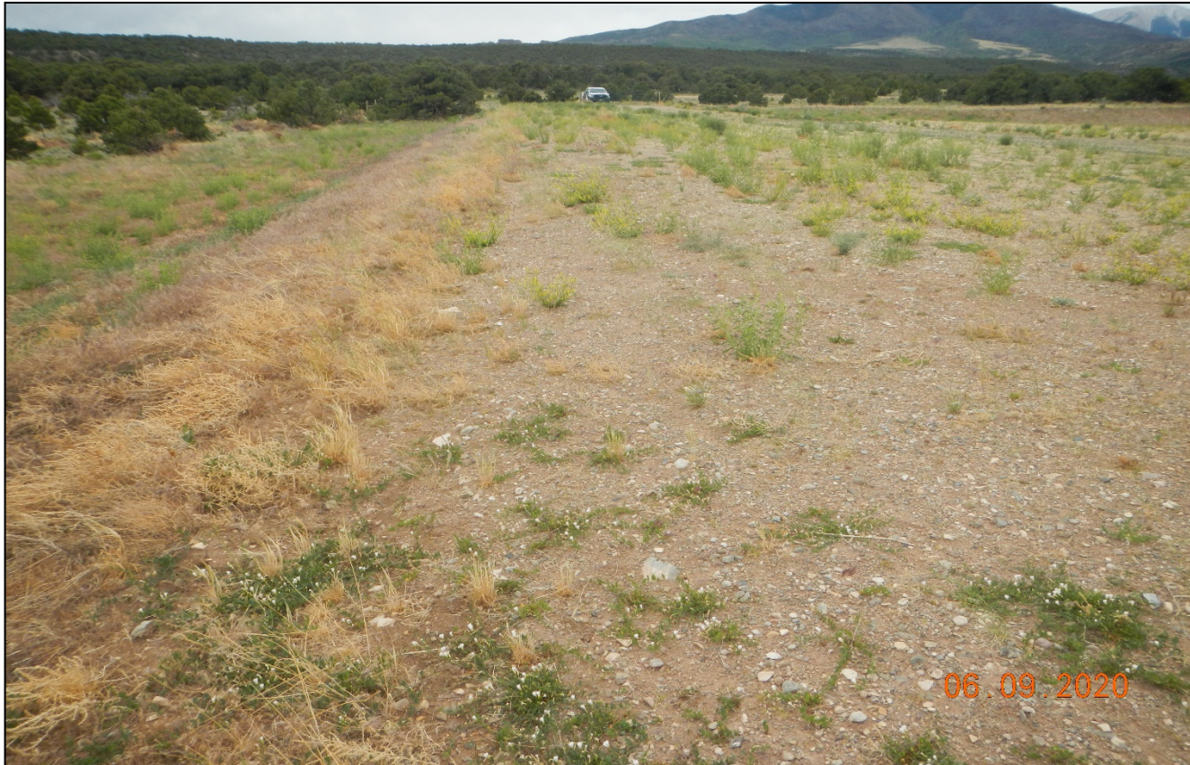
Photo 13. Facing south along the fill slope of the location. This area of the location has not been recontoured and reclaimed and gravel remains within this area.
