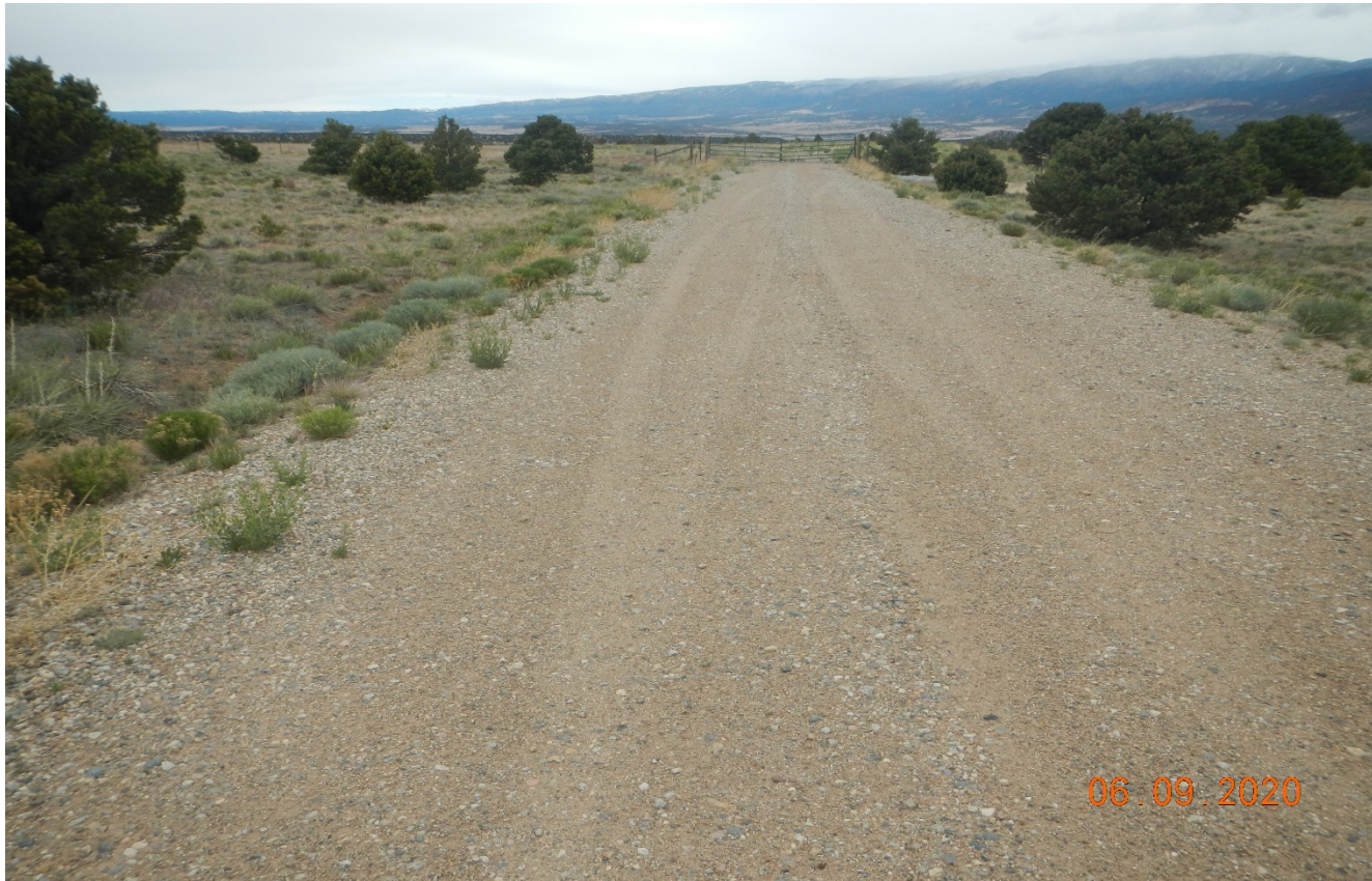
Photo 1. Facing north toward the access road which has not been recontoured and reclaimed.
