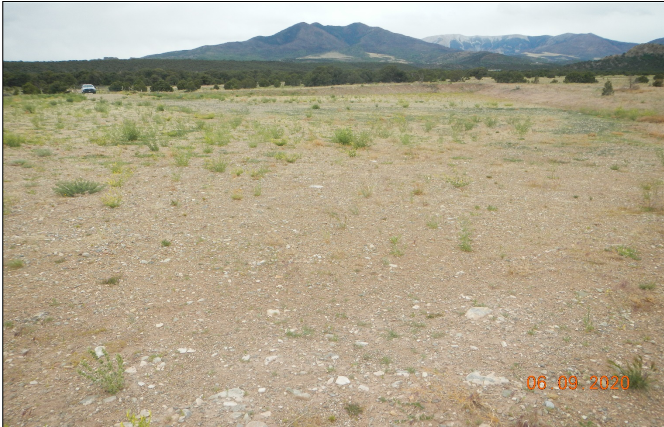
Photo 12. East side of the location facing southwest. This area of the location has not been recontoured and reclaimed and gravel remains within this area.
