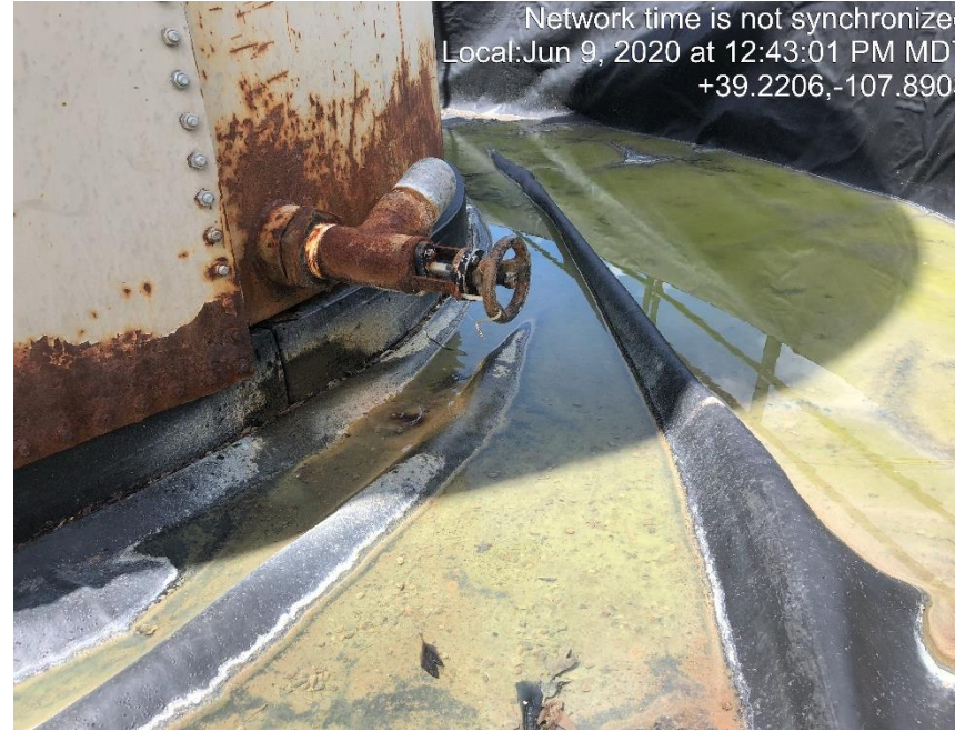
Photo #1331 Drain valve on tank #4-5 dripping condensate.
