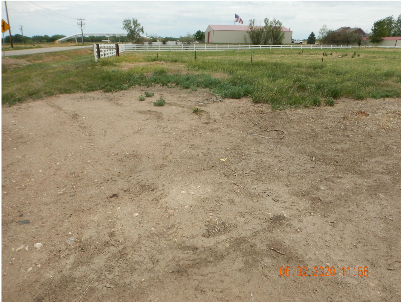
Photo 1. Photo taken from the eastern battery location, facing East. Photo illustrates all oil and gas equipment has been removed from location.
