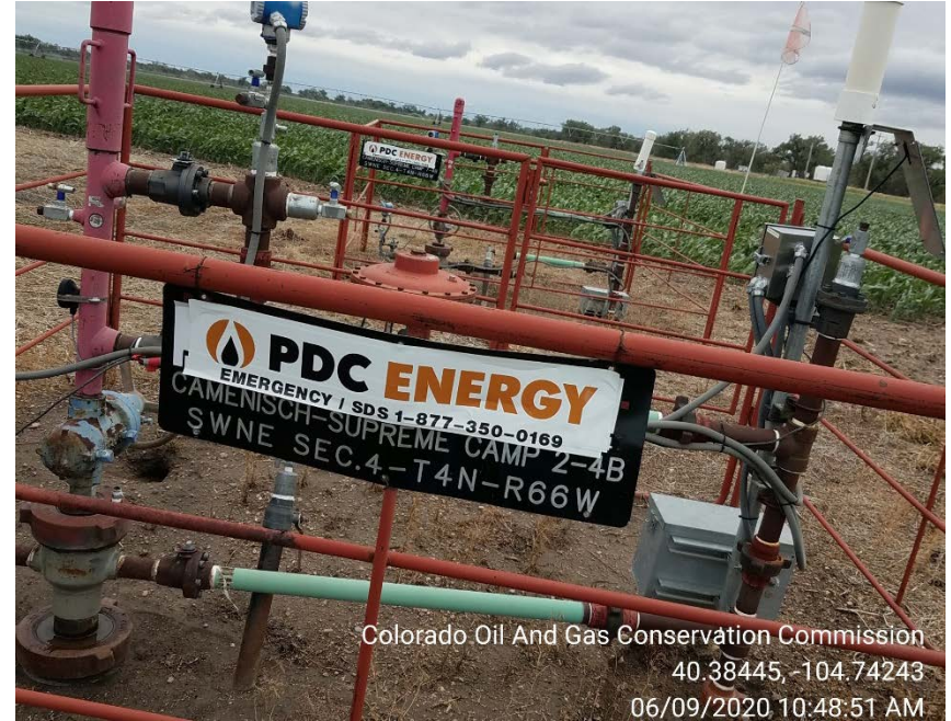
Wellhead signs on 6/9/2020
