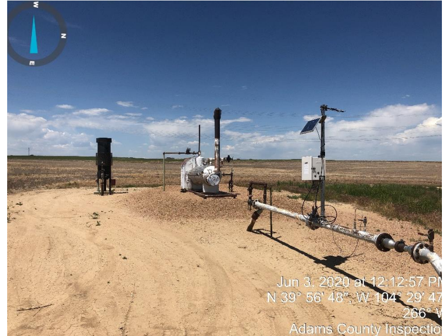
Photos #2 Meter, EDC & Separator.
