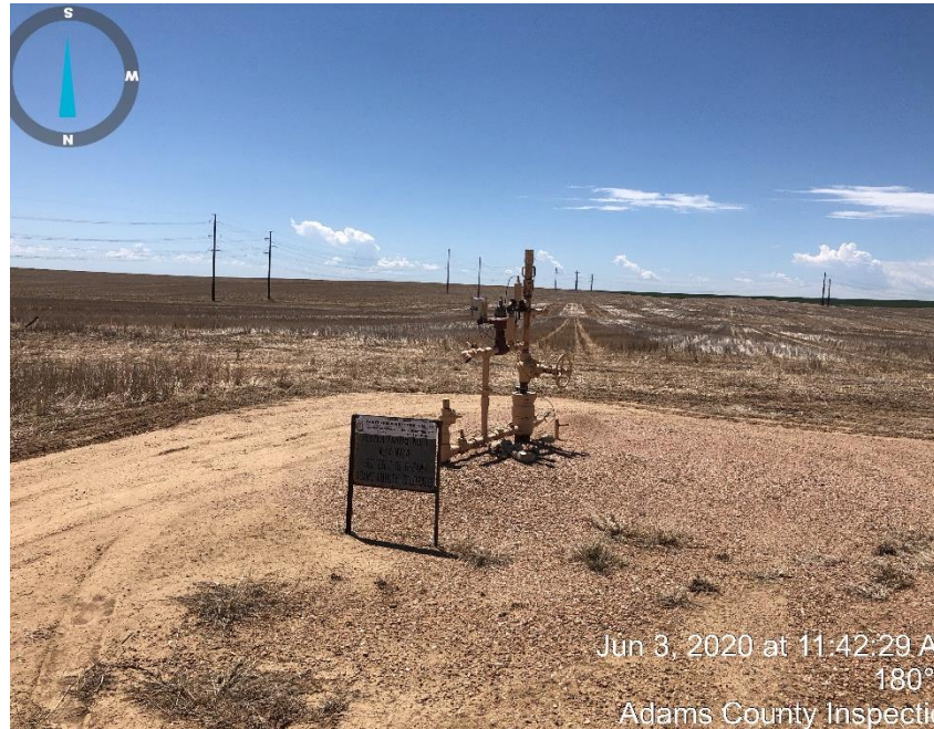
Photo #3 Well head.
