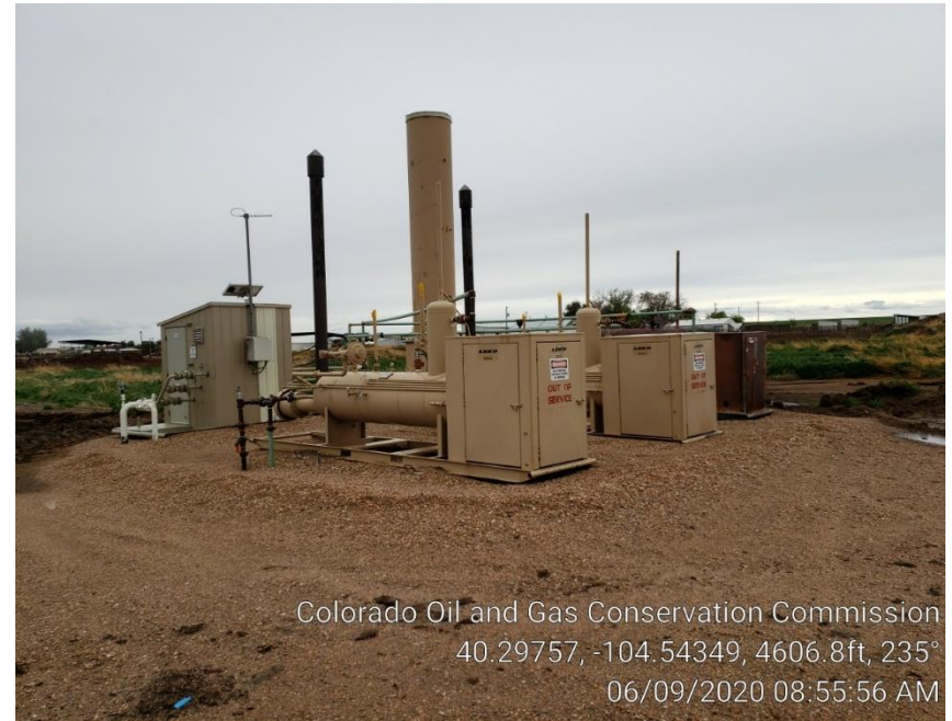
Photo #4 Separators, ECD & Meter Runs
