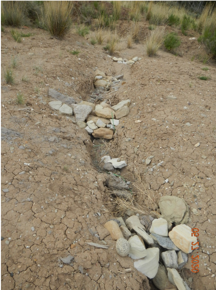
Photo#2: Undercutting of rocked checks.
