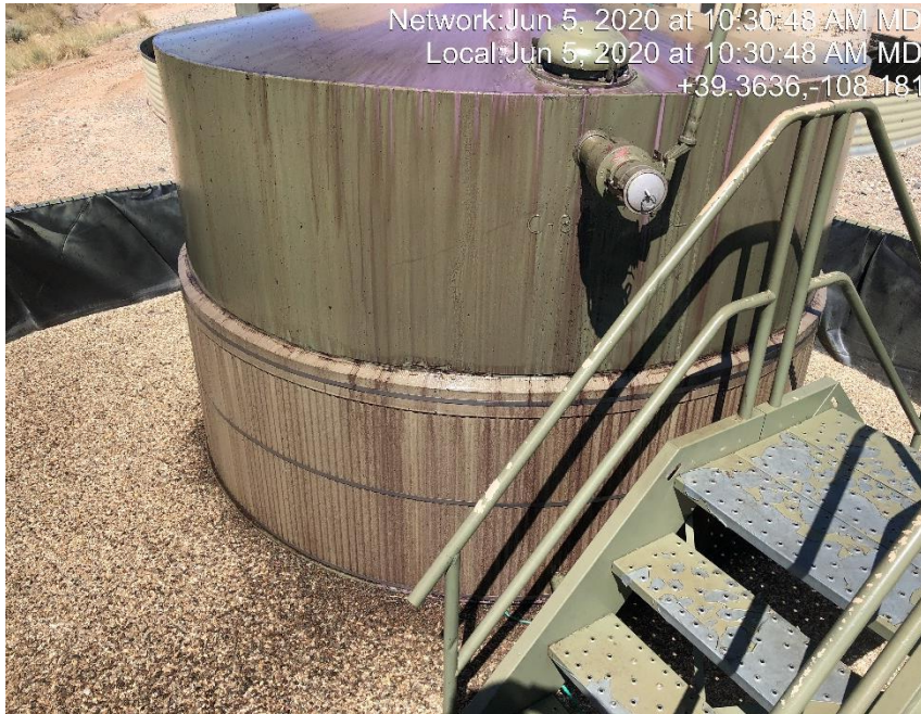
Photo #1322 Stained gravel inside tank containment.
