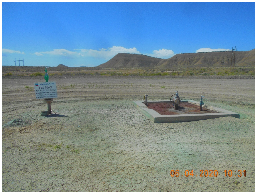
Injection wellhead. Temporarily Abandoned
