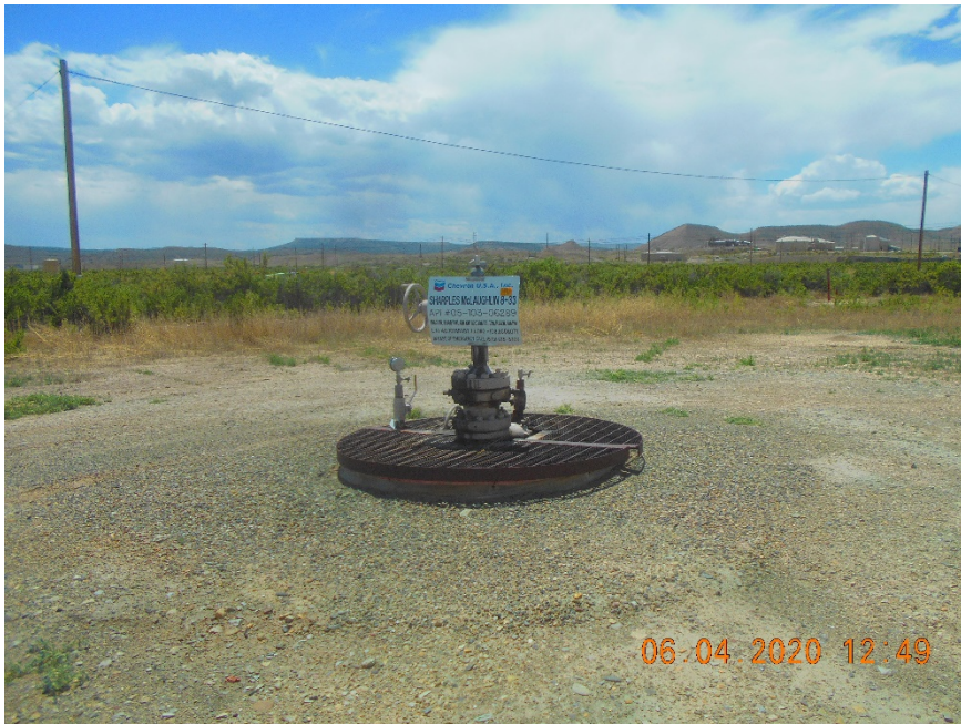
Injection wellhead. Temporarily abandoned.
